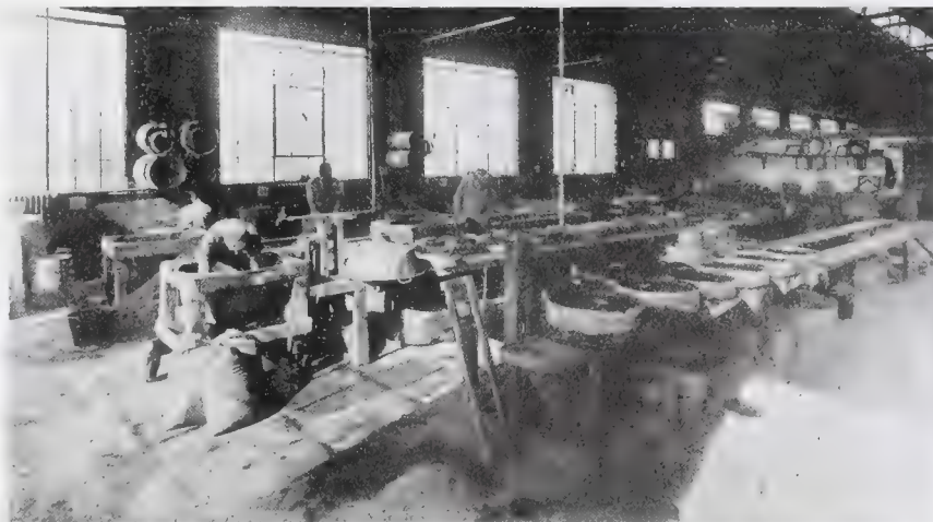
MIXING DEPARTMENT, SHOWING MIXING KETTLES AND GRINDING WHEEL MOULDS DRYING ON BENCHES. DRY-ROOM IN THE BACKGROUND.
