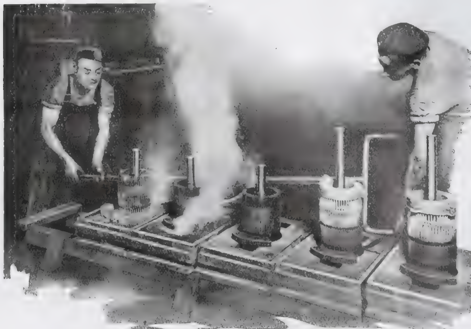
Casting End-Rings at Our Indianapolis Works.
