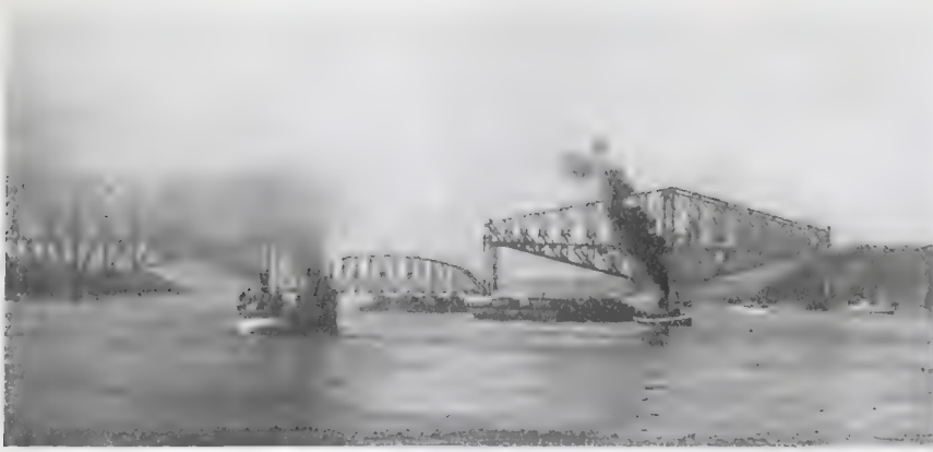
THE SPAN SUSPENDED FROM THE BRIDGE AFTER SCOWS FLOATED AWAY.
