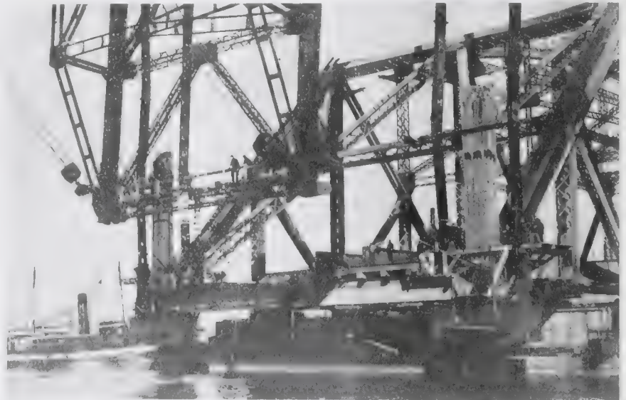
CONNECTING HOISTING CHAINS TO SPAN SUPPORTS AFTER MOORING SPAN.
