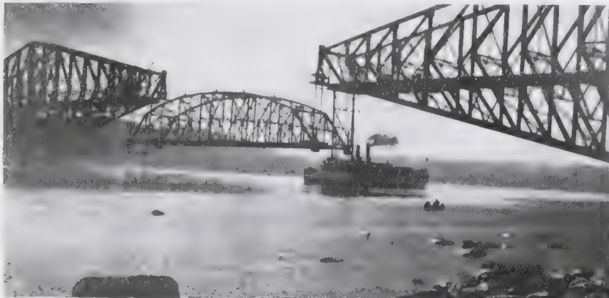
SPAN PARTLY RAISED. S.S. QUEBEC PASSING BELOW NORTH CANTILEVER.
