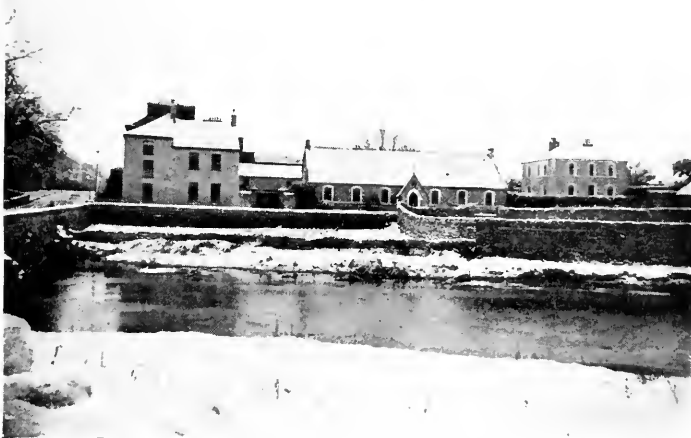
"BRIDGE HOUSE" AND BOYS' SCHOOL, DONERAILE
