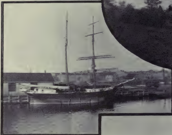
Terminal Wharf. I.C.R.
