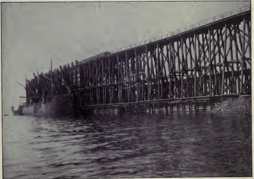
NEW COAL SHIPPING PIER, NORTH SYDNEY—NOVA SCOTIA STEEL AND COAL COMPANY.
