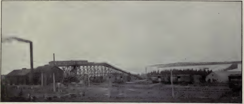
BANK HEAD, PORT HOOD COLLIERY, PORT HOOD.
