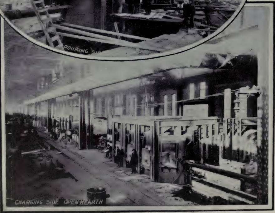
OPEN-HEARTH FURNACES—DOMINION IRON AND STEEL COMPANY, SYDNEY.
