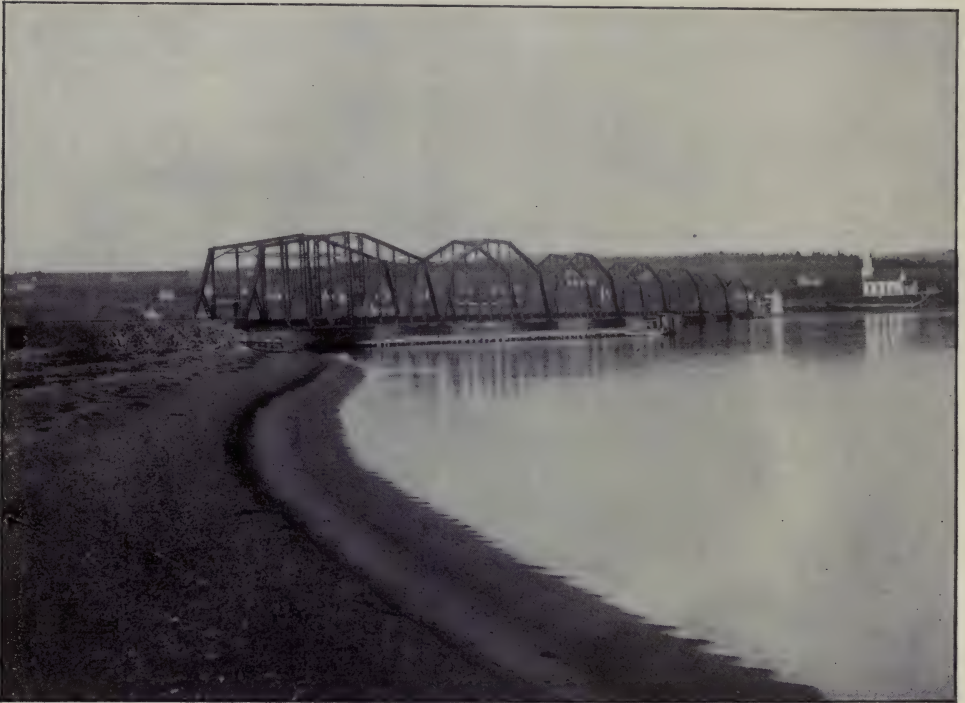
GRAND NARROWS BRIDGE, INTERCOLONIAL RAILWAY.
