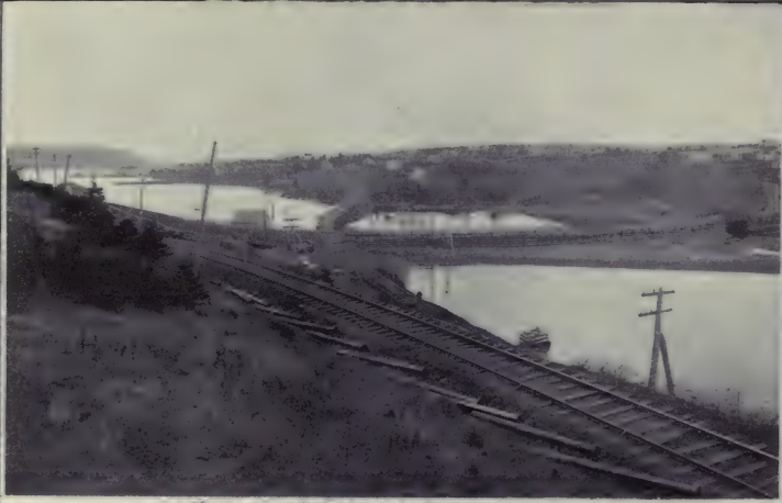
View of the Strait of Canso from the Railway and Richmond Highway.
