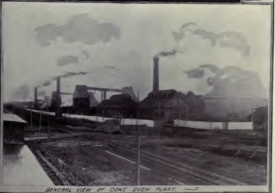
GENERAL VIEW OF COKE OVEN PLANT.
