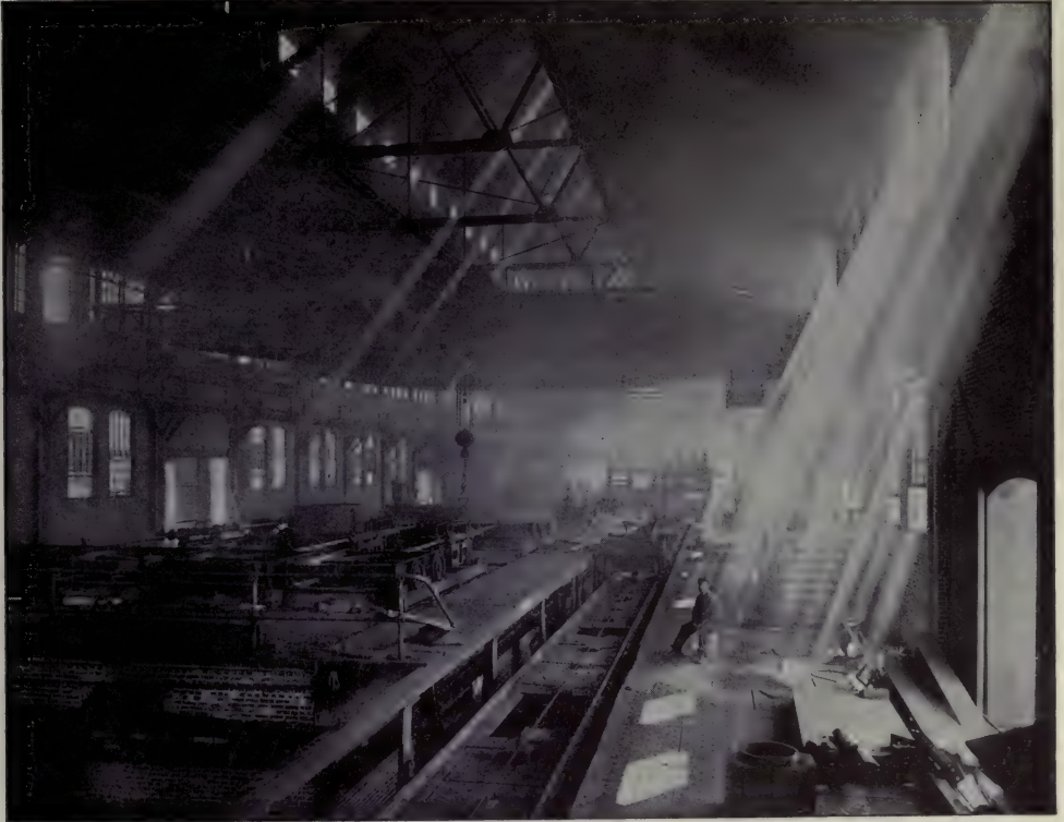
INTERIOR OF ROLLING MILLS—DOMINION IRON AND STEEL COMPANY.
