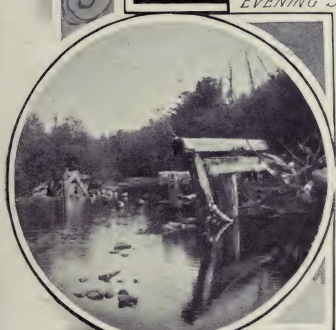
BROKEN R.R. TRESTLE.
