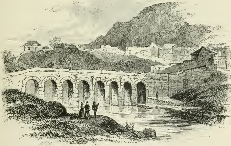
AN ANCIENT BRIDGE IN LA PAZ.
