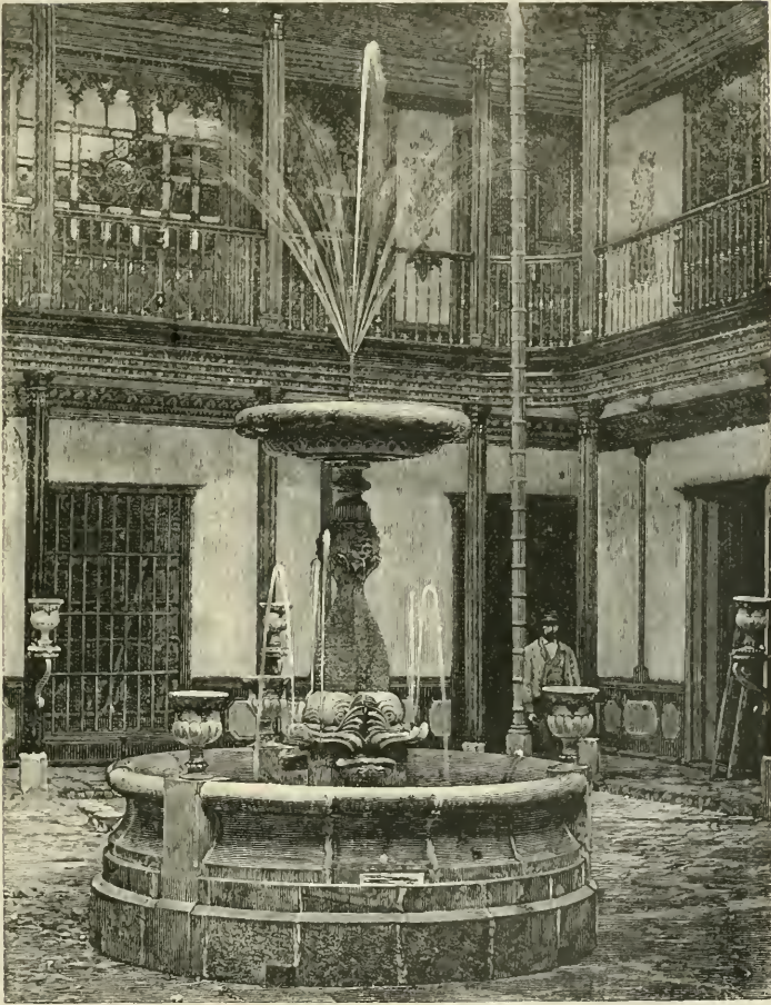
INTERIOR COURT OF A CARACAS HOUSE.
