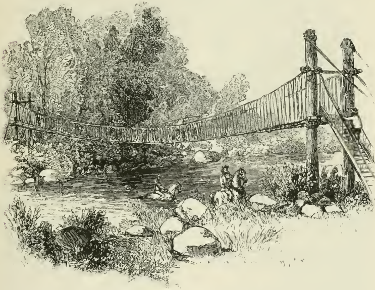
COWHIDE BRIDGE OVER THE RIMAC.
