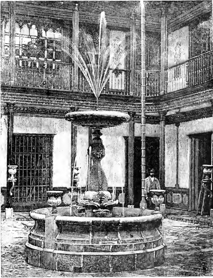
INTERIOR COURT OF A CARACAS HOUSE.
