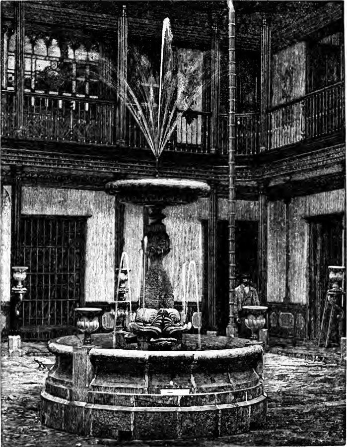
INTERIOR COURT OF A CARACAS HOUSE.
