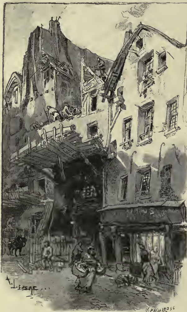
DEMOLITION OF OLD PARIS
