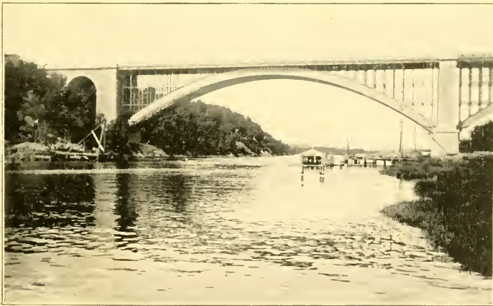
"The long arch of Washington Bridge."
