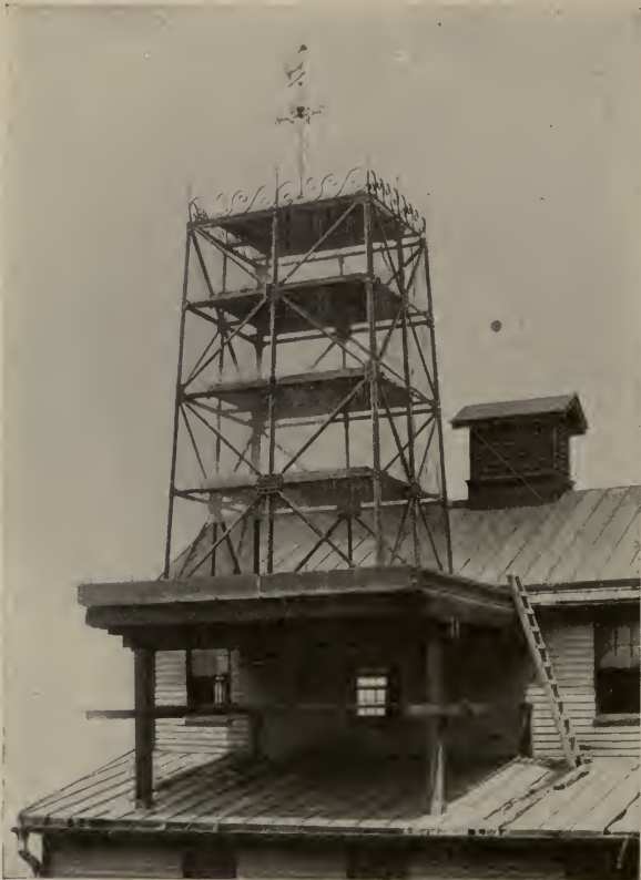
FIG. 75.—COOLING TOWER MADE OF STEEL AND GALVANIZED IRON.
