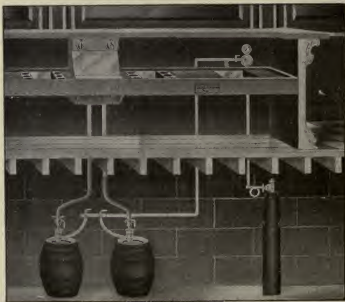
FIG. 182.—DRAWING BEER UNDER LIQUID CARBONIC ACID PRESSURE.
