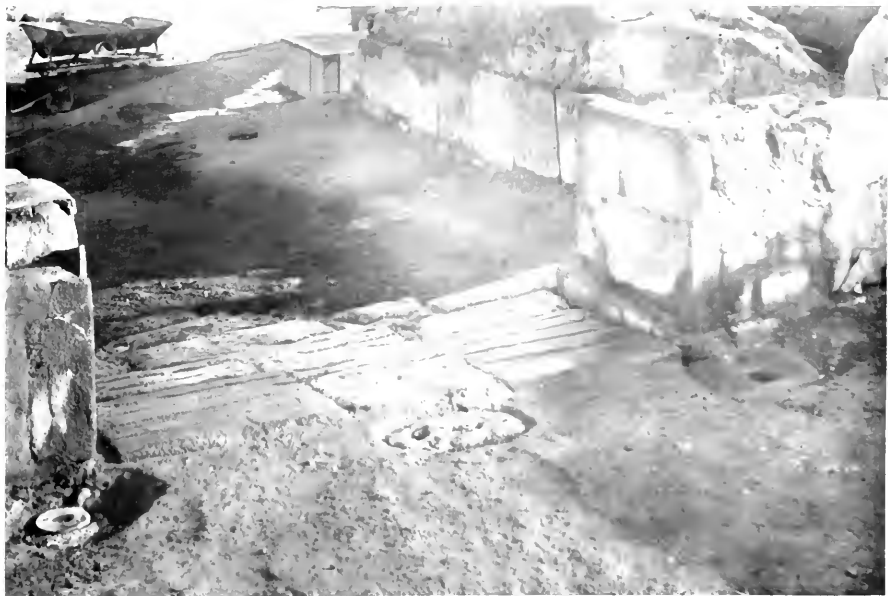
b. The outer doorway seen from inside the gate-chamber, showing the grooved threshold, the two basalt slabs of the nearer part of the threshold, and the inscribed slab (A. 9. 2. 1. A. 12)
