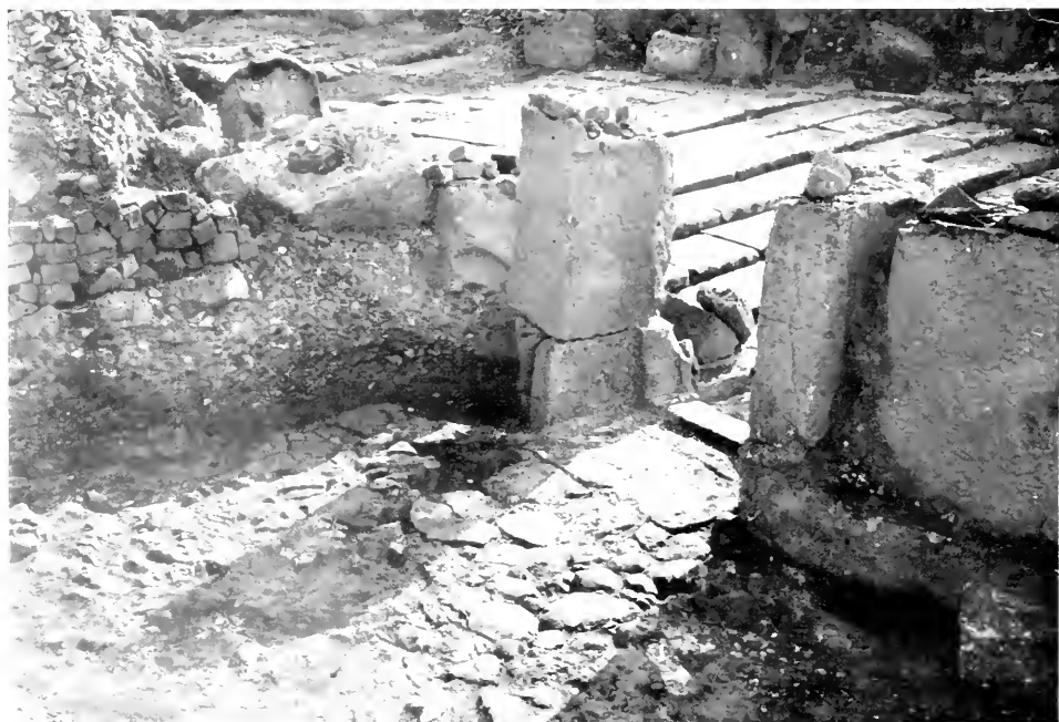
b. The door on the Staircase seen from inside the West Passage, after the replacing of the south jamb
