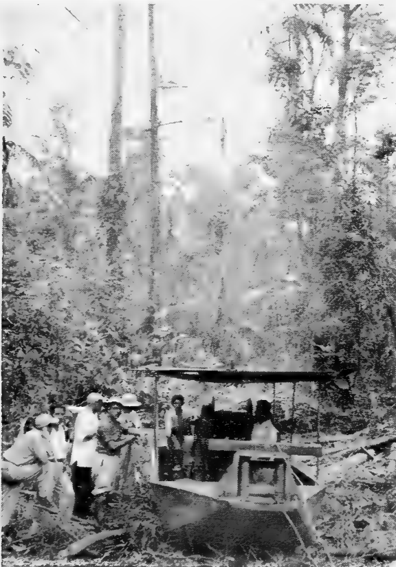
Figure 4. - Double drum winch mounted on barge in the "guandal", used to drag cuangare logs from the guandal to stream banks.
