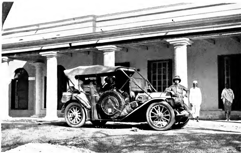
A Dāk Bungalow at Burdwan, Bengal, India. One of the Government rest houses
