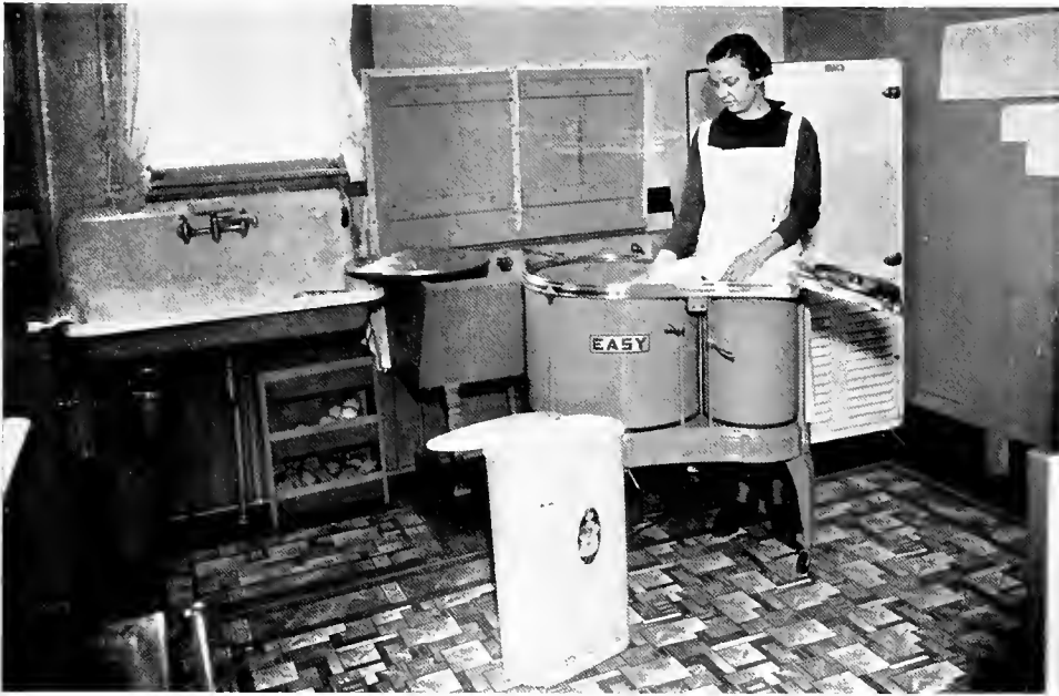
Modern Laundry Unit
