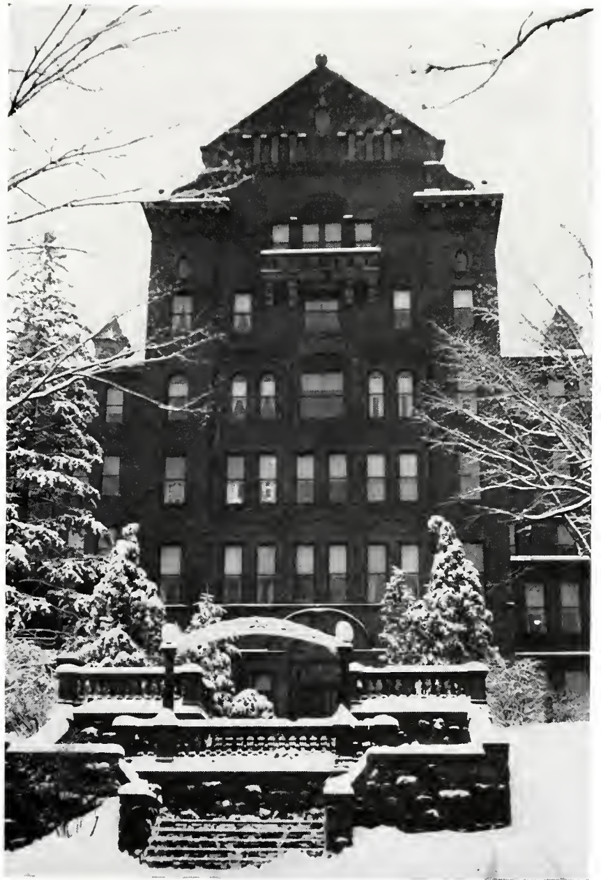
NORTH HALL ENTRANCE .
