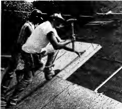
ThermaCal being applied to the roof of a residence in waferboard sections.
