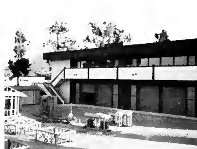
VENTURA COUNTY, CALIF. — This JATC dedicated its new training center last November. There were 55 apprentices in the first PETS class. Ventura county was an early supporter of PETS.
