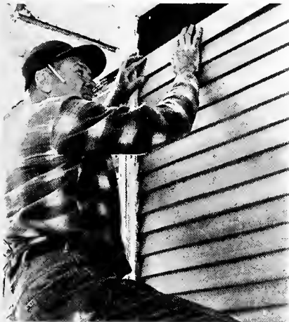
Art Burke scrutinizes some of his siding alignments on the Reagan home.
