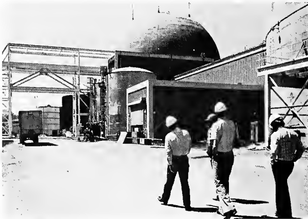
When labor editors, including the Carpenter's associate editor, went through VEPCO's North Anna facilities near Mineral, Va., last summer, only North Anna 1 was operating. Its reactor dome is seen in the background. North Anna 2, meanwhile, was left idle so authorities could check false fears expressed by environmental groups that the plant was on an earthquake fault.
