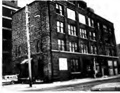
DES MOINES, IA. — This JATC recently purchased and is renovating a four-story building as a training facility. All 23 fourth-year apprentices are expected to complete PETS this year.
