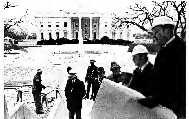
Ken Ritchey, president of Associated Builders, Inc., contractors, looks over the work with Frank Fields, vice president; Donald Simmons, secretary; and Robert Graulich. With them from the General Services Administration were Ross Lawson, Richard Super, and Robert Weppner.
