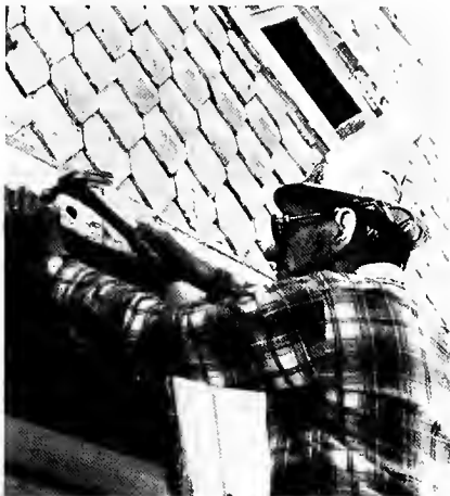
Howard Glenn wields a hammer in the restoration efforts.
