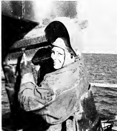
Laurie O'Gara of Local 1456, New York City, prepares for a welding job aboard ship. She is a dockbuilder and holds a commercial diving certificate.
