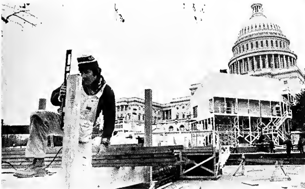
Dale Menestrina of Local 1590 aligns an upright as he works on a railing for a spectators' stand.
