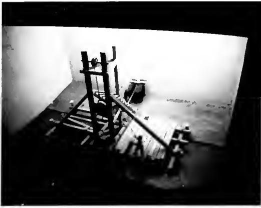
LEFT: A museum model shows the pile driving methods of the early Egyptians, as two oxen, background, lifted a heavy stone into position to be released by the man on the platform. Heavy logs were floated down the Nile to assemble the rig.
