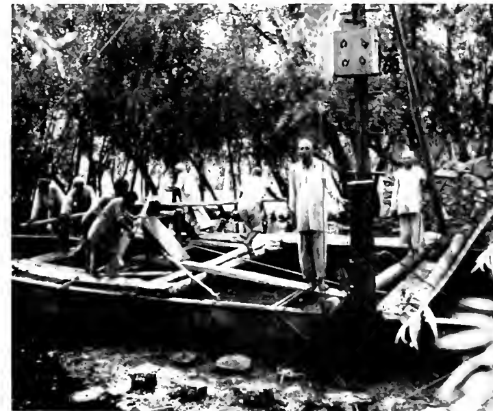
ABOVE: This primitive rig, using manpower alone, is still in use in rural Kashmir, India, today. Note the piles in foreground, already set in the soft topsoil.—Photograph by Luke Golobitsh of West Germany.
