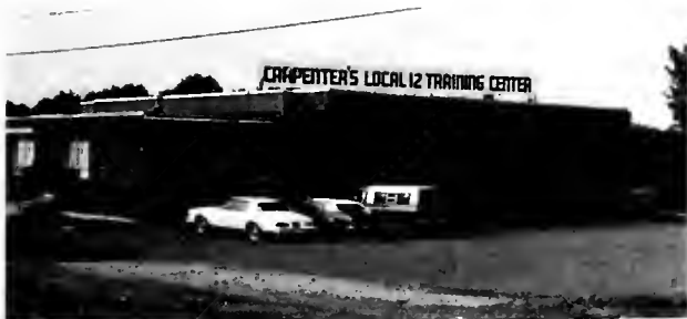
A former American Freightways terminal remodeled
