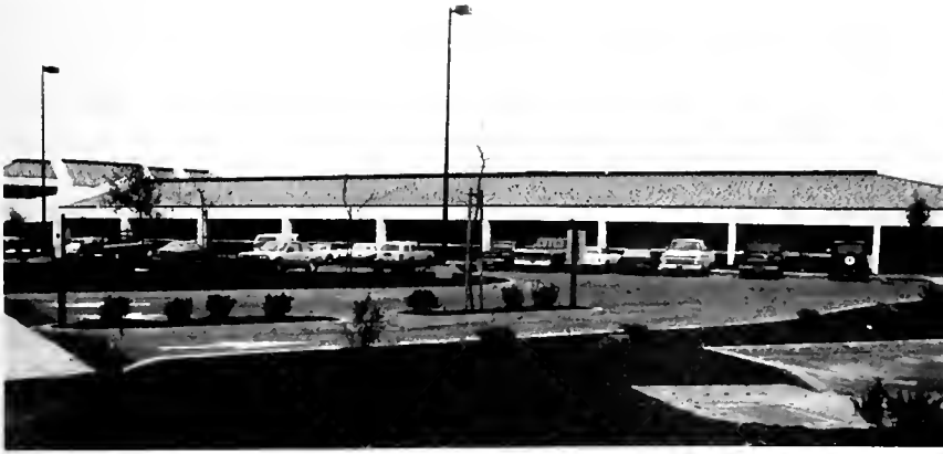
Classrooms of the Carpenters Training Center face Santa Rita Road, Pleasanton. The two-story building in the background contains administrative offices and the supporting service of training material development and production. Adjoining shop areas are used for manipulative instruction and laboratory practice.
