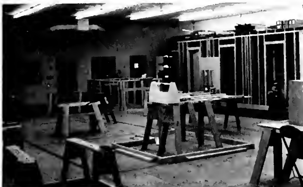
Interior view—of the new Syracuse work area.
