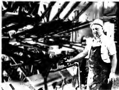
Gus Burns, Local 94, puts some edge-glueing through the glue wheel.
