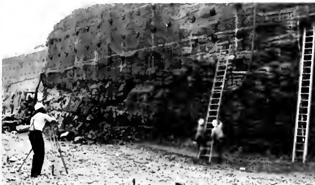
Foundation work continues at the site.
