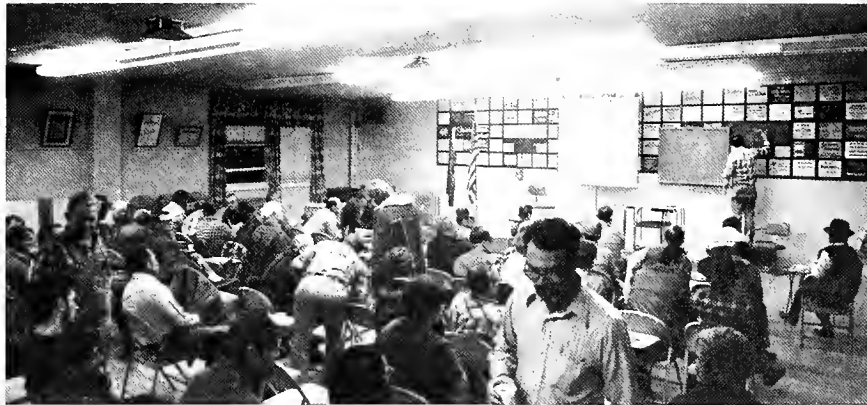
It was almost a "full house" at meeting hall in Lewiston, Idaho, as journeymen assembled to learn the ways and means of erecting concrete grain elevators, using the slip-form system.
