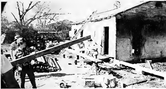
Local 213 members begin renovation on the Mack home in northeast Houston.
