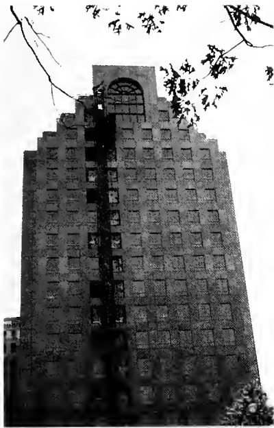
The Fleet National Bank building framed by the Providence sky.
