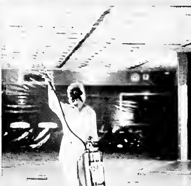
Photos, clockwise, from top right, show worker holding a piece of asbestos insulation; spraying asbestos insulation with a wetting agent in preparation for removal; pipes with sprayed-on asbestos insulation; proper enclosure of a ceiling with asbestos insulation.
