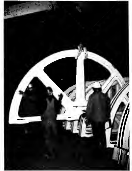
Foreman Don Foster of Local 102 watches half of a sheave wheel being hoisted into place.
