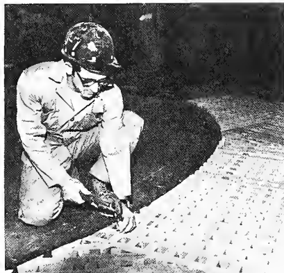
Rylee and Ross insert the last section of grating, testing for proper fitup prior to installation aboard ship.
