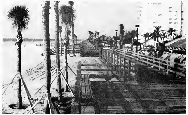
The boardwalk has about 24 covered areas with benches for people to sit and relax at intervals along the beach.
