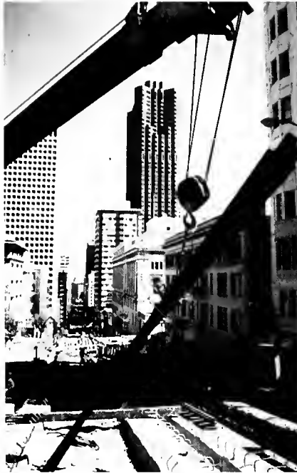
Foreman Don Foster of Local 102 watches half of a sheave wheel being hoisted into place.
