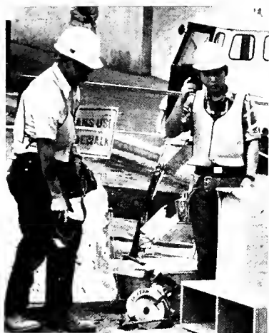
Apprentice Carpenter Rosemary Leyson of Local 483, San Francisco, works on building the forms for the concrete pour at Powell and California Streets.
