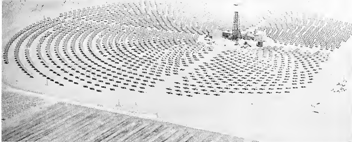
The Solar One Pilot Plant—an array of 1,818 mirror modules, called heliostats, which ring a 298-foot receiving tower and reflect the sun's rays toward a boiler unit atop the tower. The resulting steam is piped to a turbine and generator below. The steam is condensed, cooled and returned to the boiler. The 10 megawatt plant was built by UBC millwrights and other construction tradesmen on 130 acres of California desert.
