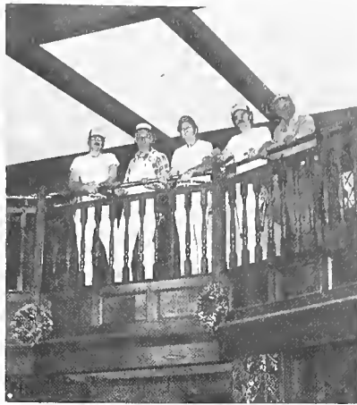
Carpenters who installed the new staircases in the Henry VIII Inn's lobby are, from left: Mike Evrard, Bill Hunch, Gil Nash, Gary Evrard, and Bob Evrard of Ellisville Enterprises, Inc. All the visible wood is oak supplied by shops and mills under contract with the CDC. The carpet was installed by members of Floorlayers Local 1310.—St. Louis Labor Tribune photos
