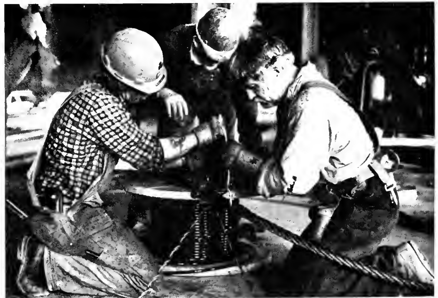
Local 102 Millwright Stan Boren works on splicing the cable as the ironworkers reeve it.
