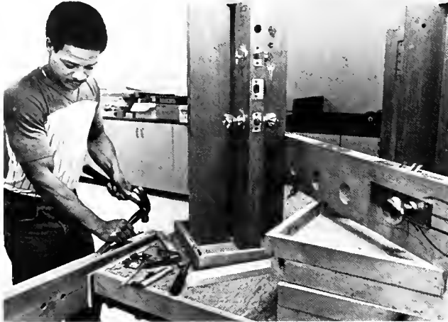
Apprentice Darryl Plummer mortises a door butt in Detroit's lock installation class.
