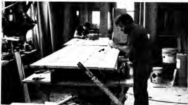
Barry N. Hahn, foreground, and Kenneth W. Wehr Jr., background, work on doors to be installed in the U.S. Department of State's Diplomatic Reception Rooms.
