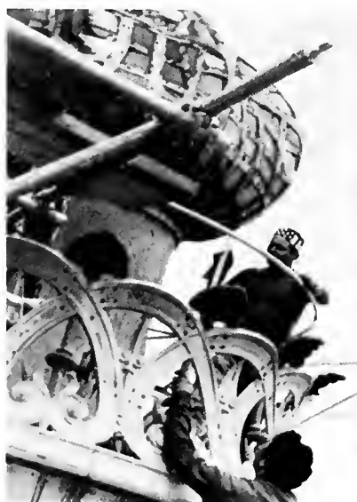
Several attempts have been made over the years to light the torch from within by cutting out sections of the copper and using various types of lighting. In the end, Bartholdi's original intent was the best; the new torch replicates his design of a copper flame with 24-carat gold-leaf. At left, Elnut Leonardello, Local 1536, helps prepare the old torch for lowering. Photos © Dan Cornish/ESTO.
