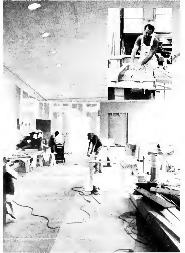
The job foreman, Randy Payne, Local 132, Washington, D.C., is shown on the upper level of the East Building working on the exhibit sales area while Tom Piddington, Local 1665, Alexandria, Va., insert, works downstairs in the exhibit shop.
