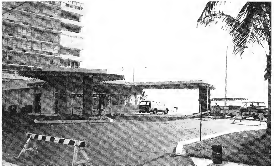
The newly refurbished Voyager Sightseeing Train station.
