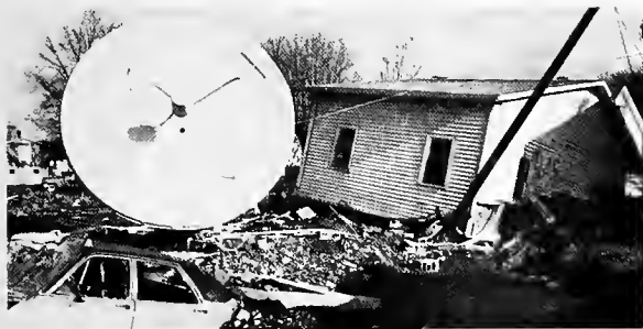
A house tilts crazily and a car lies half buried under debris in the aftermath of the flood which devastated Moorefield, W. Va., last November. The number on the building designates it as condemned and scheduled for removal.—National Geographic Society photograph
