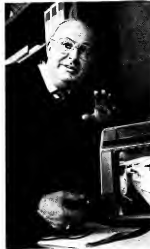
Instructor Cicero Haralson advises Stanley Kuznicki on the proper use of a power plane. Power tools are used only after hand tools are mastered.—Photographs by The Detroit Building Tradesman.
