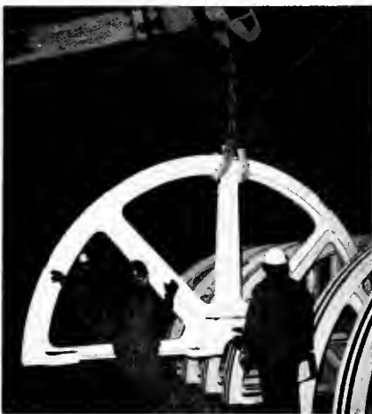
During the 1984 restoration of the cable cars in San Francisco, Calif., hard-hatted workers installed the sheave wheels.
