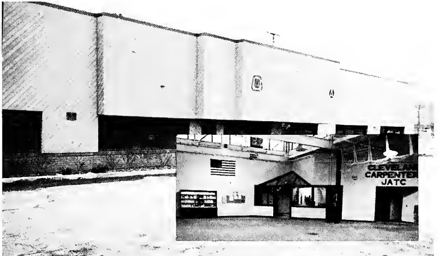
The Cleveland apprenticeship school is pictured above; inset shows center of operations.
