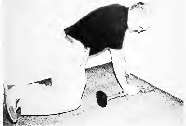
A carpet layer, right, demonstrates the knee kicker. Below right is the power carpet stretcher, a "knee-saving" device.
