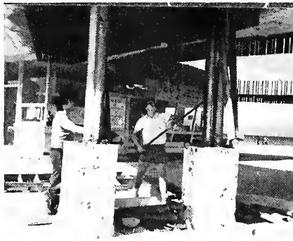
VOC Chairman Mike Decker and State Organizer Gordon Long work on the demolition of the old facade.
