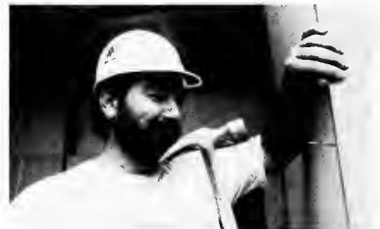
Brian Bailey, Local 906, Glendale, Ariz., looks pleased to be pounding another nail in place for this community service project.
