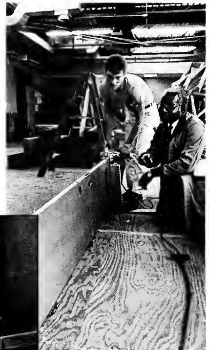
Instructor Cicero Haralson advises Stanley Kuznicki on the proper use of a power plane. Power tools are used only after hand tools are mastered.—Photographs by The Detroit Building Tradesman.
