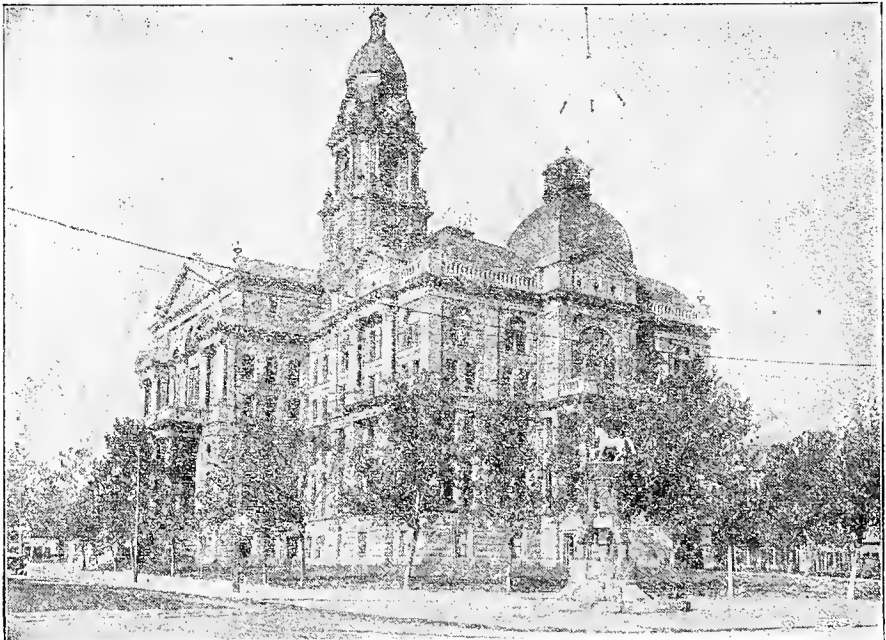
Tarrant County Courthouse.
