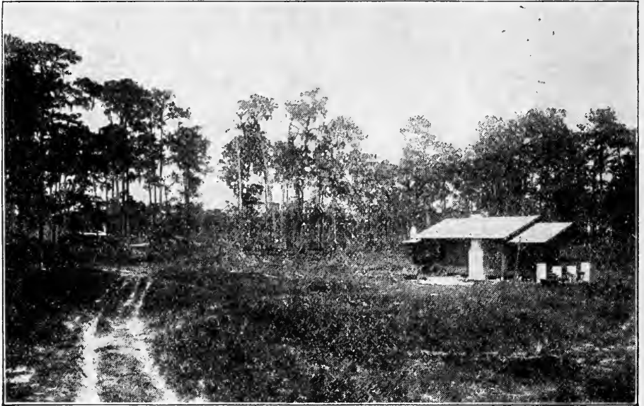
View of Land Under Development On Site of the Home For Our Aged Members, Lakeland, Fla.
