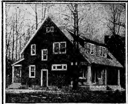
Residence of Walter M. Collins, Builder, Bayside, L. I.
