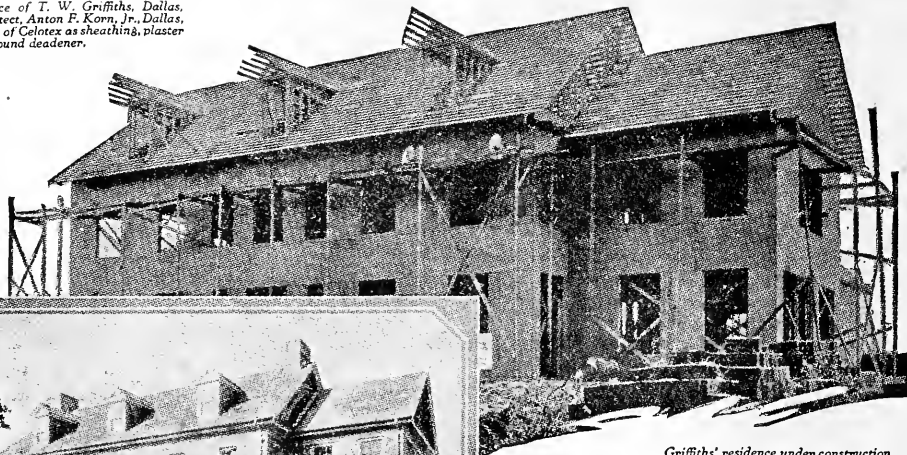
Griffiths' residence under construction showing Celotex applied directly to the studs in place of wood sheathing.
