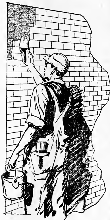
A coating of white or ivory enamel makes it glisten like real ceramic tile
