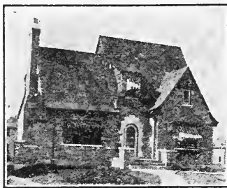
One of the hundreds of homes attractively and durably roofed with J-M Asphalt Shingles.
