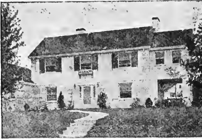
House in Kansas City, Mo. Architect Edward Buchter Delc. Insulated with Cabot's Quilt. Painted with Cabot's DOUBLE WHITE. Roof Stained with Cabot's Creosote Shingle and Wood Stains.
