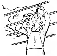
Nail furring on 16' centers, right over old plaster.
