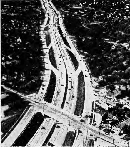
Urban portions of Interstate System now being built under 13-year highway program will look something like this. Divided heavy-duty roadways of two or more lanes will carry express traffic over or under intersecting streets without stoplights. Bordering service roads will collect and distribute freeway traffic safely and efficiently.
