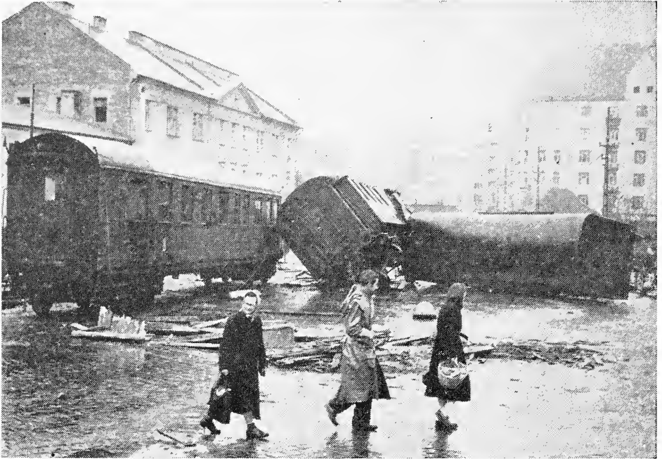
Mute, but graphic evidence to the violence of the fight that occurred in Budapest are these overturned railroad cars in the city's South Station.— World Wide Photos, Inc.
