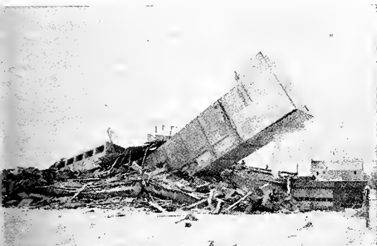
Six-story 70-unit lift-slab apartment building—almost ready for occupancy when the quake hit. The intact portions are the stairwell and the elevator shaft, which were poured-in-place reinforced concrete.
