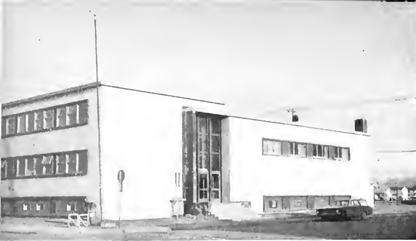
Poured-in-place reinforced concrete. Undamaged by the quake. The building is plumb. The flagpole used to be.
