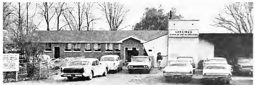
Lansing's School of Special Education is at right, above, and the new sheltered workshop is at left. Cars of workers from the Chicago Building Trades Council fill the yard, as skilled craftsmen applied finished touches to the interior of the new workshop. The building measures 70 by 34 feet and would normally cost more than $45,000 to erect.
