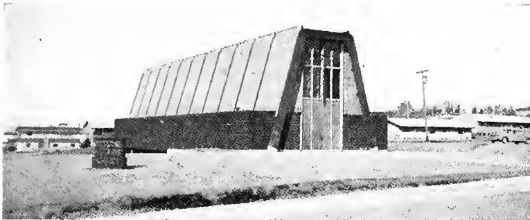
All wood structure on reinforced concrete foundation. No damage.
