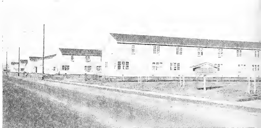
Federal low income housing project—150 units—wood frame construction (650 kids). Damage—one concrete block central chimney.
