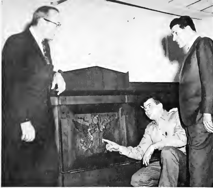
Admiring a finished rostrum for the Rayburn Office Building in Washington, D. C. are, left to right, Jerome B. Lande, president of George Weiss Company; Thomas Paone, shop foreman; and John Anello, Metropolitan District Council business representative. Each of nine eagles in the center of committee rostrums was hand-carved in solid walnut.
