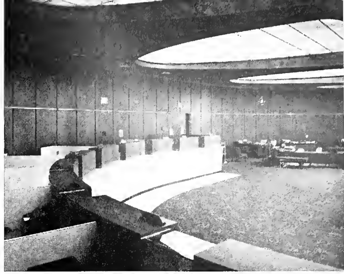
WILLIAM M. McVEIGH won praise “for excellence in placing of the grounds in the main banking room of the Riggs Bank’s Lincoln Branch. It was a complicated procedure, because the room was oval-shaped, and the panels were installed with concealed fastenings. Grounding out for this job was considered by the judges to be as important as the finished surface.
