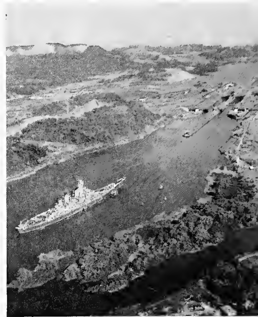
This aerial view of the present Panama Canal suggests the lush, tropical jungle through which construction would be pushed. A naval dreadnaught prepares here to negotiate narrow passage.
