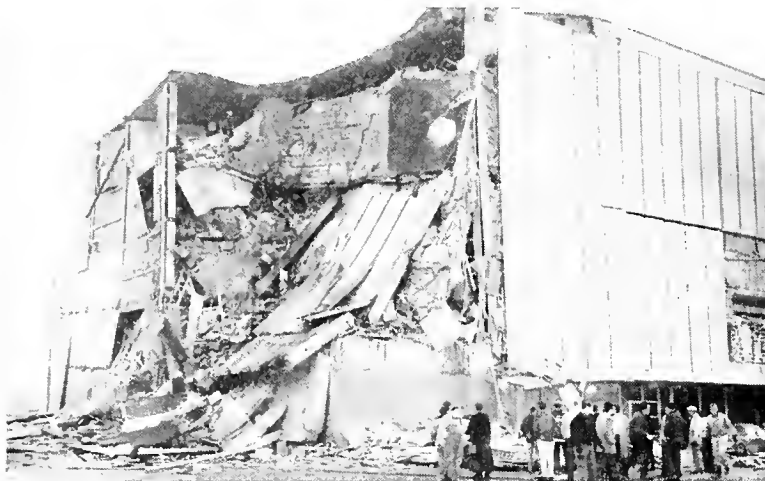
Concrete slab curtain wall. Couldn't take it.
