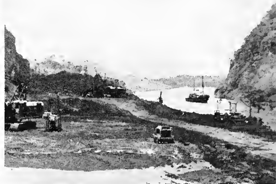
Intermittent widening operations have been carried out by the Corps of Engineers throughout the Canal's brief history. Here the Gaillard cut is widened by 200 feet in 1960 operations.
