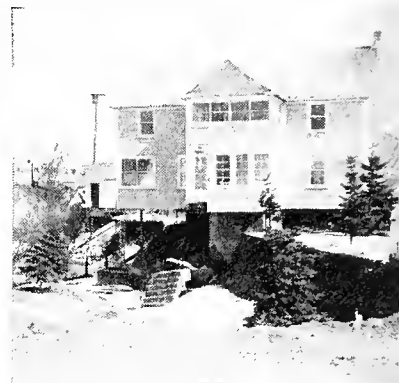
A new foundation is all that is needed here.
