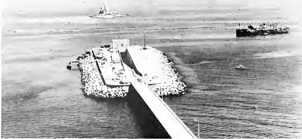
Man-made islands provide entrance into the mile-long tunnel under Thimble Shoal ship channel. Each island is a quarter-mile long and covers eight acres at the surface of the water. Sand was pumped from the bay bottom by dredges to form the core of the islands. Heavy stone armor protects against storms. The islands are built in 35 to 45 feet of water and rise an additional 30 feet above the surface.
