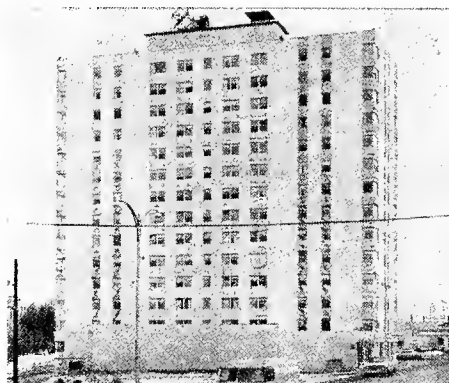
14 floors of poured-in-place reinforced concrete. Battered but not beaten.
