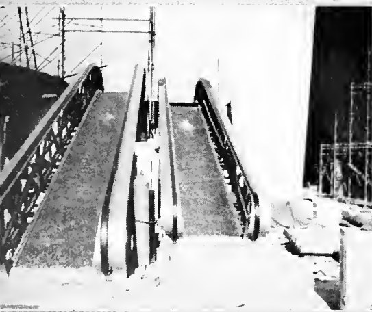
Two speed ramps at the Gas Pavilion, shown at left, are examples of work by Millwrights and Machinery Erectors. They lead to a Pavilion turntable.
