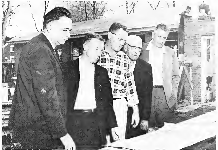
Project Coordinator, work supervisor, and prime mover in the erection of a sheltered workshop for a school for the handicapped in Lansing Community, Illinois, was George Vest, Jr., center above, business representative of the Carpenters' District Council. He is shown here conferring with representatives of other unions, including, from left: John Boland of the Plasterers, Jim Hamilton of the Lathers, C. O. Muffitt of the Painters, and Peter Herberg, business agent of the Painters.
