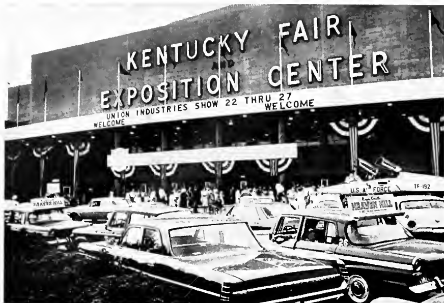
The Kentucky Fair and Exposition Center at Louisville was decked in bunting and fluttering pennants for the AFL-CIO's big 1964 extravaganza. People, taxis, and private automobiles crowd the entrance to the exhibition hall in the view at left. More than 200,000 persons passed through the gates.
