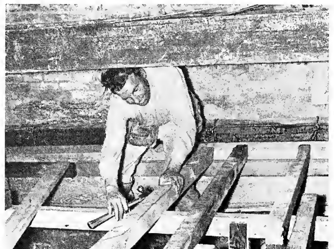
Wayne Dye, Local 528, works on a deck.
