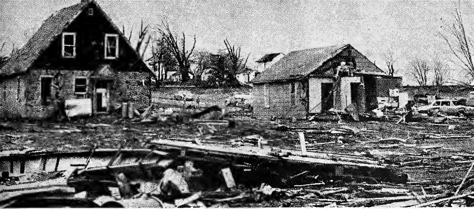
While no structure is safe from tornado damage, some well-constructed houses have sustained comparatively little structural damage in the midst of chaos.
