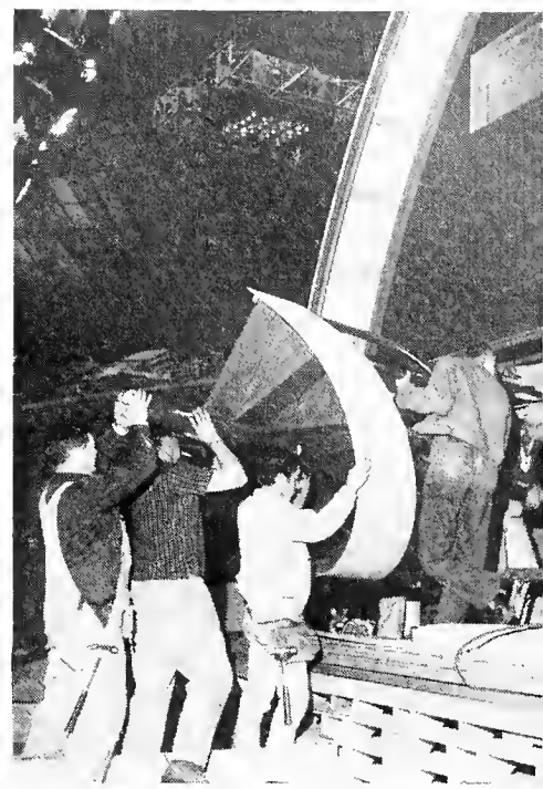
Carpenters move a spiral stairway into a one-room Olympic "Shal-A".
