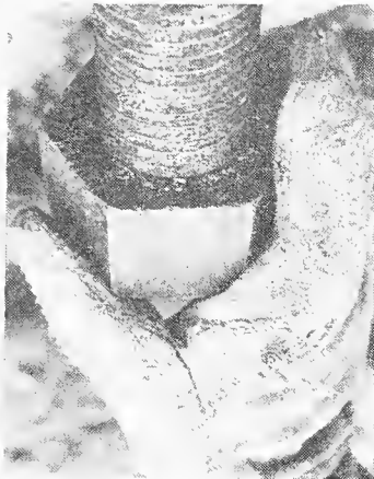
A skilled, gloved hand applies a nut to a big tie rod.
