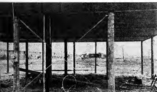
RIGHT: A pole-type house can be attractive as well as sturdy. BELOW: Cable cross-bracing adds rigidity without offering resistance to waves. Also note good practice of plywood sheathing under the house for added protection.
