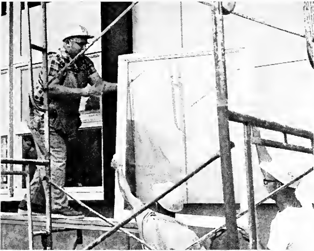
Installing one of 700 wood-framed windows in pilot plant.
