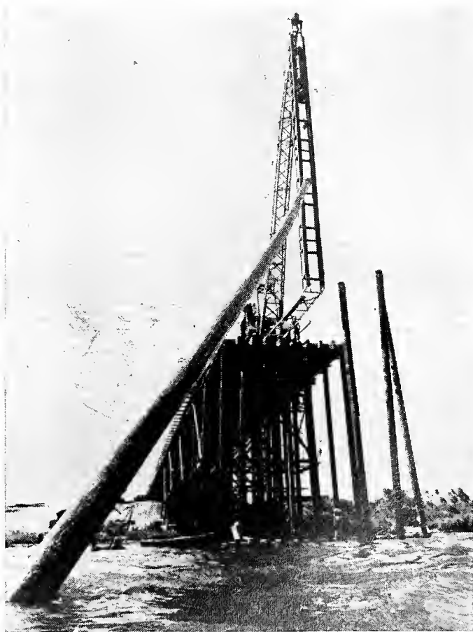
PILE COMING IN —An 85-foot piling is moved into position for driving. Seven of these piles were each driven 20 feet to support the roadway, 32 feet above the river's low-water level. In all, 800 piles were driven into the river bottom to complete Liberty Bridge.
