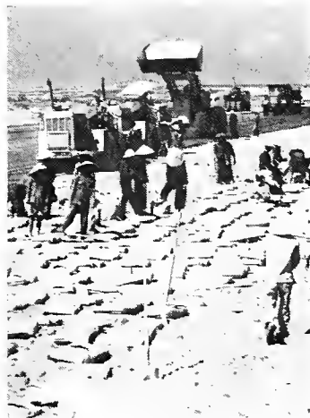
Construction staple in Vietnam is the familiar bulldozer (left) shown here crossing sand to tow supplies from landing ship docked at waters edge. Vietnamese laborers (center) distribute bags of cement as they prepare a soil-cement base of aluminum runway matting. Local labor helps erect pre-fab buildings (top right), and (below right) a sketch entitled "Roof-tops, Danang," where one of our northernmost bases is located. Sketches by Marine Corps Capt. John T. Dyer. Defense Department Photographs.
