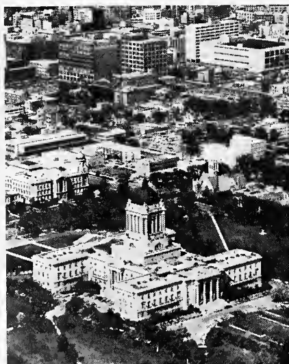
Manitoba's Legislative Building is said to be one of the most beautiful parliament buildings in North America. Seen from the air, its magnificent architectural design and its almost sylvan setting in the heart of Winnipeg, can be appreciated.
