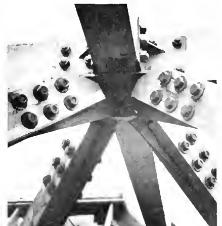
Steel connectors were designed to tie in Douglas fir laminated beams with bolts. Pricing found steel system 30% higher than wood. High sales potential is seen in commercial, industrial fields, where heavy timber rating is advantageous.
