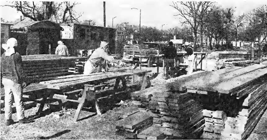
Local 14 members at work in the Guido Brothers construction yard.
