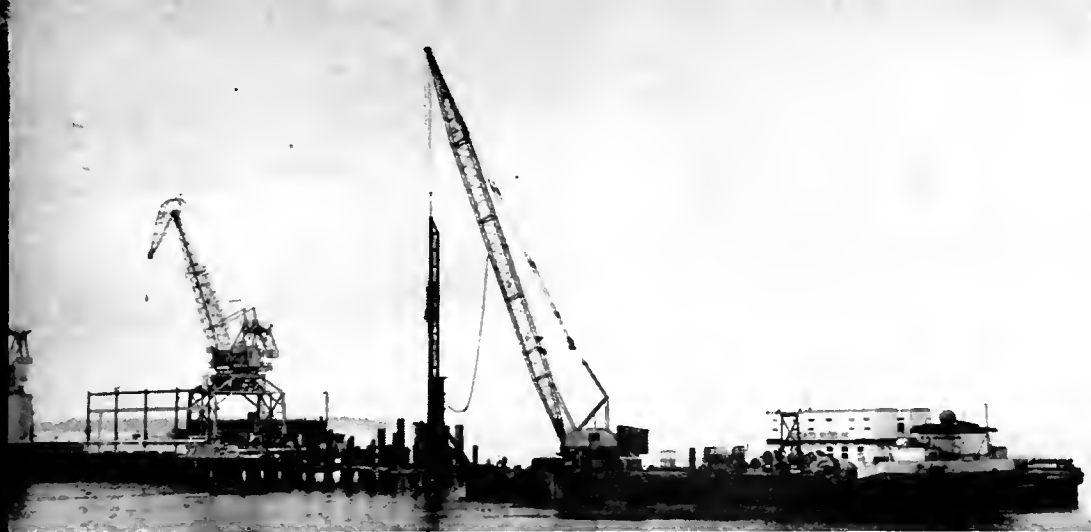
An overall view of the barge-mounted piledriver at work on the dock extension. Six lines anchored the work barge as the work continued at a steady pace around the clock.
