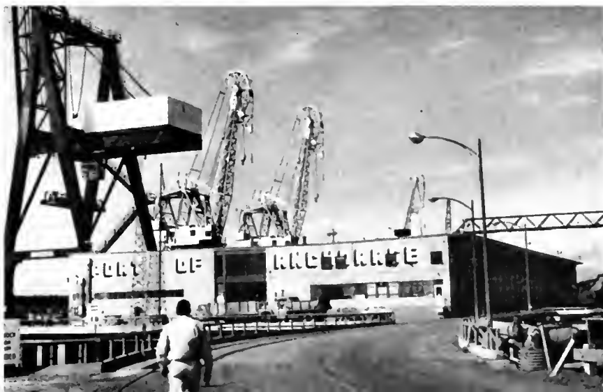
Below: The port facility at Anchorage can berth ships of up to 20,000 tons and will handle two ships at a time when the dock lengthening is completed.
