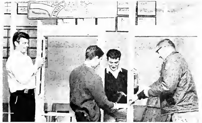
Three trainees installing the rough framing for window and door openings and fire-blocking.
