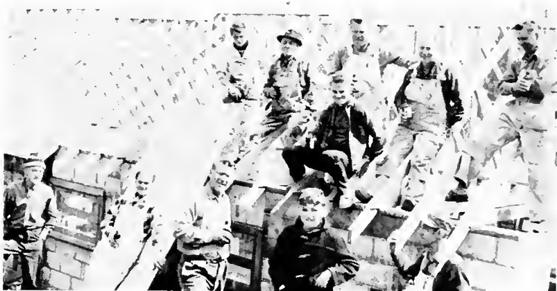
Members of the Brotherhood take a break from their work of completing new toilet and washroom facilities at the Jubilee Camp. This was one of many work parties.
