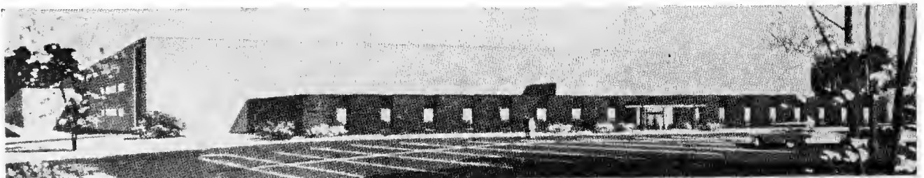
The 140,000-square-foot plant south of Battle Creek, Mich., where Levitt Building Systems, Inc. has begun its first modular homebuilding operation. The assembly line at this plant is expected to turn out colonial-style townhouses to sell for $20,000 to $25,000 (with land) plus models for Operation Breakthrough (See Pages 8 and 9). The Tri-Trades Label at upper left, combining union labels of each of the three unions, is to appear on each new modular home produced by Levitt.
