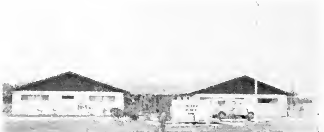
A view of the Osceola Children's Home as seen from the entrance. The home is located in Orlando, Fla., and was built by union labor.
