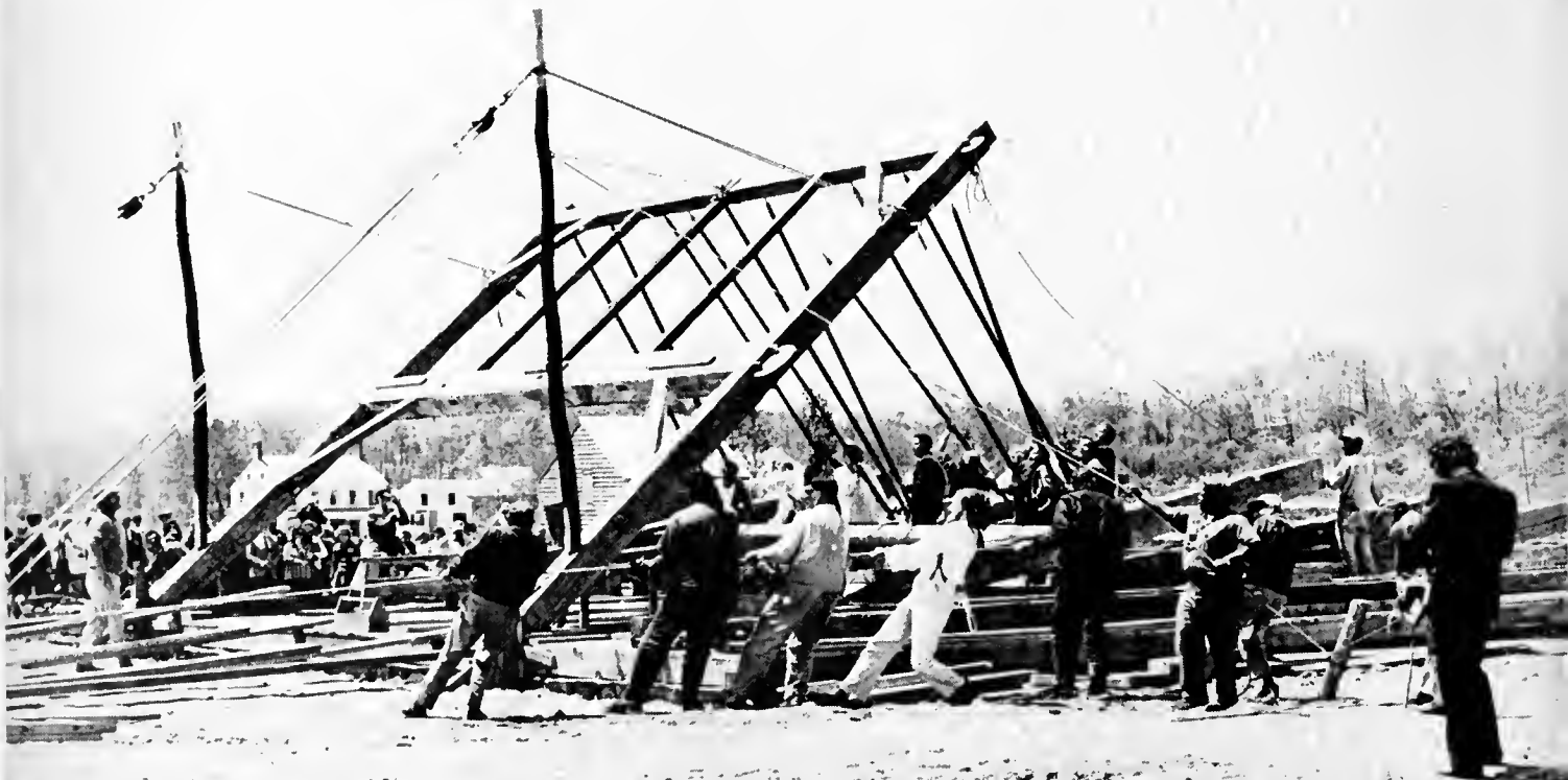
The first section (called a bent) weighed 2½ tons and required sturdy backs to pull into place. Note pre-stacking of bents.
