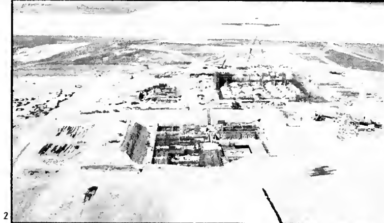
3. The "blanket-covered" northwest corner of the Perimeter Acquisition Radar Building. Sheets of plywood and Styrofoam cover concrete curing at 50-degrees F temperature, despite below-zero outside temperatures.
