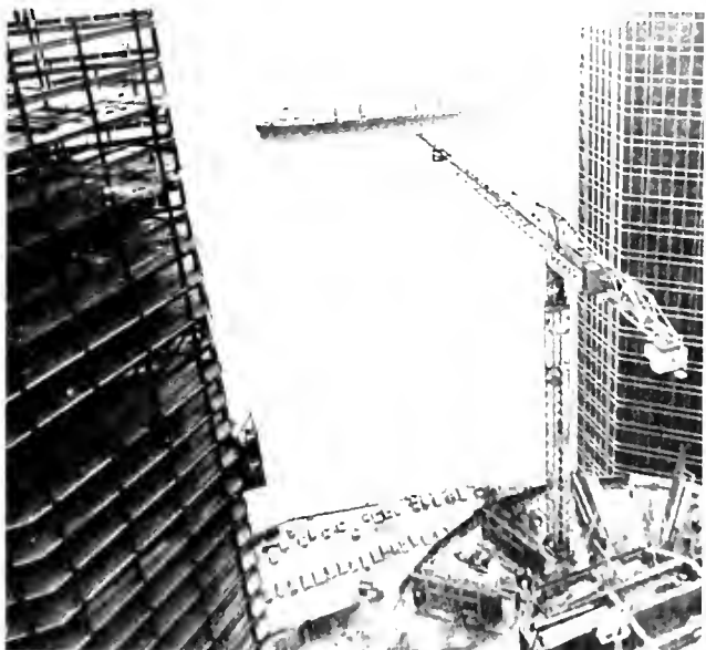
One of the famous longboats which ply the Detroit River with their cargoes of iron ore moves past the towers of Renaissance Center. The tallest tower in the center rises 719 feet above the street. The center is constructed mostly of reinforced concrete, and carpenters have completed as many as two floors a week on some of the buildings in the complex.
