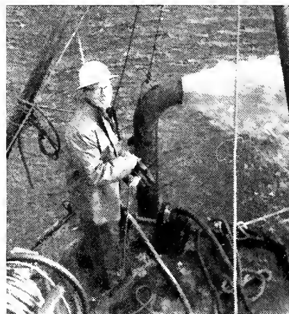
A tender checks the flow of sand and debris from an air siphon, as his diver works below.
