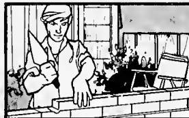
Lay brick with speed and precision!
