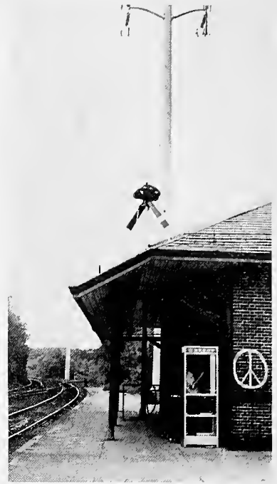
The Needham Railroad Station near Boston, Mass., was originally built about 1850. An outdated peace symbol still marred one section of brick wall, as the roof was braced for repairs.
