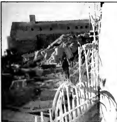
Pictures below were taken last fall, as winter came on. High winds twisted the iron rods in the concrete forms during the night. At lower right, a Building Tradesman checks the lines on an ice-crusted crane.
