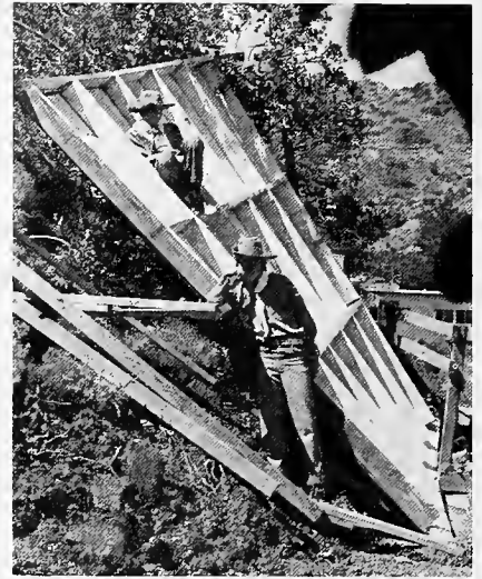
Scouts survey the damage done to Cherry Valley Boy Scout Camp on Catalina Island.
