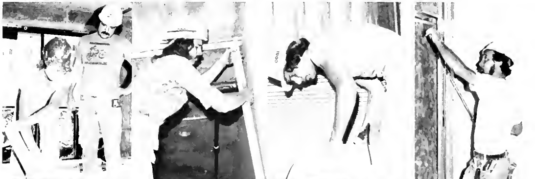
TOP ROW: From left, Karl Johnson, job superintendent, watches son, Blaine, cut drywall; Apprentice Steven Bain installs a partition; Willie Frunhenberger of Local 132 at work; and John Garcia on metal framing.
