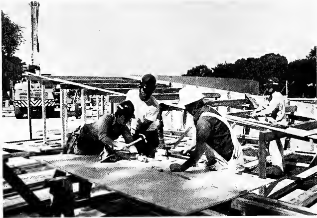
Washington, D.C., members prepare a massive outdoor altar for Pope John Paul II's Mass on the Mall. In the foreground are Apprentice Nancy Meyer, Local 1590; Ken Reed and Francis Hardesty of Local 132.
