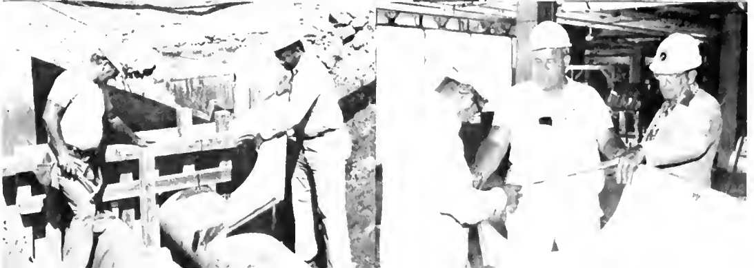
BOTTOM ROW: From left, Frank Beavers of Local 1665 and Calvin Braxton on form work; and DC Business Rep. Jim Merkle, right, with Bob Jones, Buck Field, and a plastic-laminated column.
