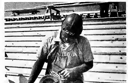
Robert Oliver of Lake Forest, Ill., notches one of the more than 500 stringers with a Skil saw.
