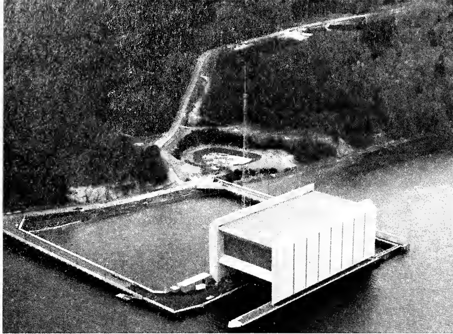
Explosives Handling Wharf No. 1, equipped to load and unload missiles under cover.
