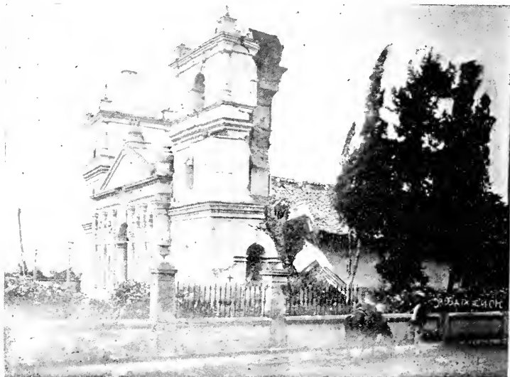
The Church of Our Lady of the Angels. It was a famous earthquake resisting building, but this time failed.
