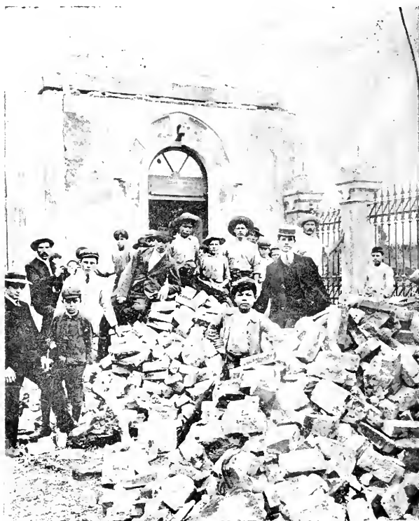
Almost a total wreckage at the Municipal Slaughter house in San Jose, after the earthquake of April 13th 1910.
