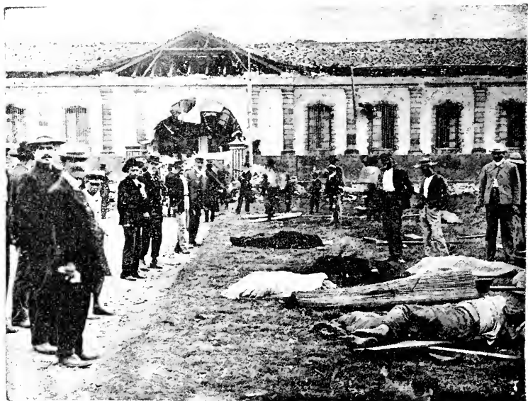
Bodies of people killed by the earthquake waiting identification in front of the ruined Armory House.
