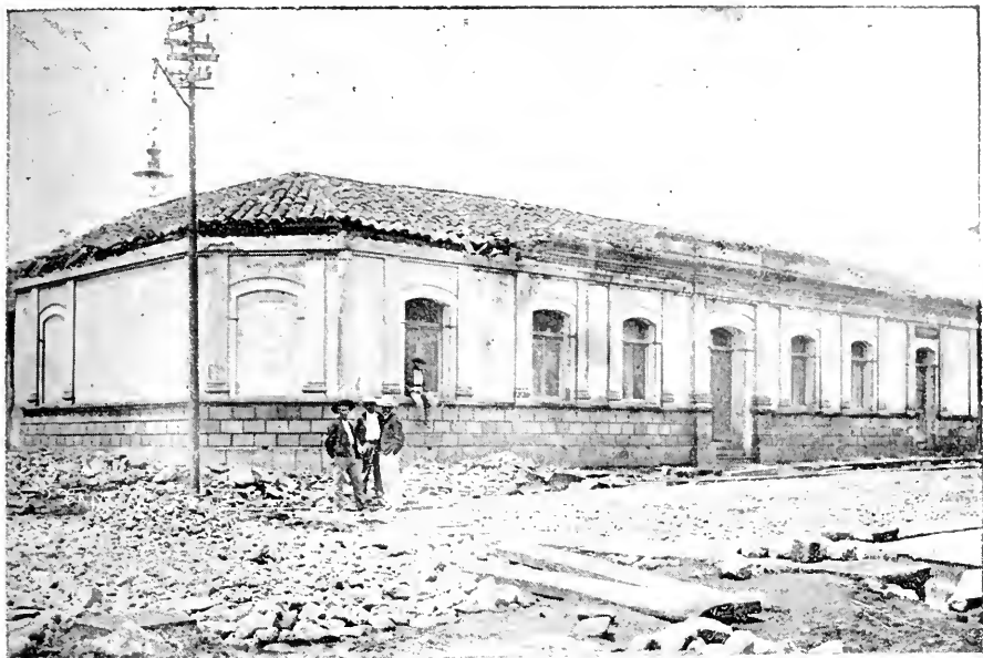
How the buildings at Cartago withstood the earthquakes just before the fatal shock.
