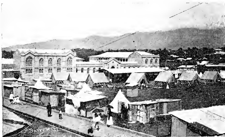
A view from the Mercedes Plaza in San Jose, facing the San Juan de Dios Hospital (undergoing extensive earthquake repairs). Those tents erected are the gift of the American Red Cross who responded nobly to the appeal made by President Taft.
