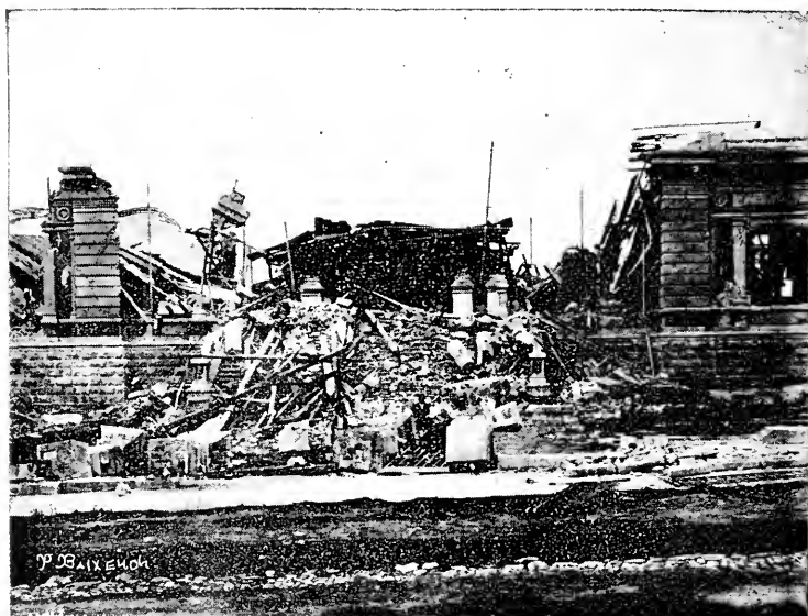
A view of the Central American Court of Justice, after the shock. This Palace constructed with the gift of $ 100,000-00 donated by Hon. Mr. Andrew Carnegie, was nearly finished.
