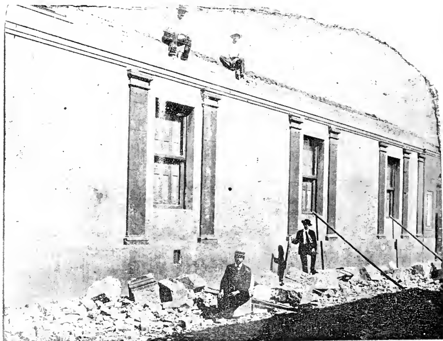
One of the residences in San Jose almost wrecked, after the earthquakes of April 13th 1910.
