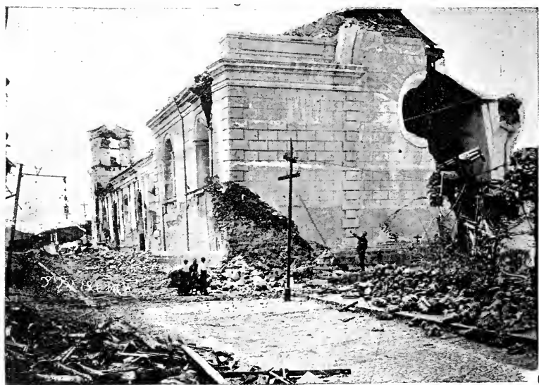
Back of the Church of «La Soledad» as it was seen the morning after the earthquake.
