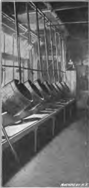
Fig. 2. Tubs used in Washing the Cups after Annealing
