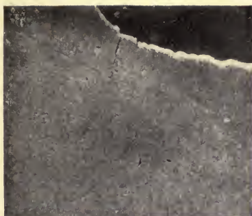
NO. 52. AT EDGE OF SHELLED-OUT SPOT.
