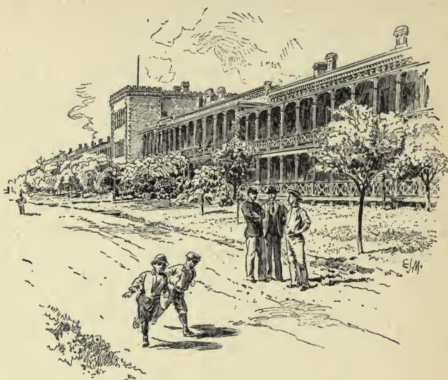
THE BARRACKS, FORT HOUSTON
