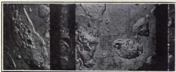
FIG. 60.—Phosphide blisters on cemented gear.
