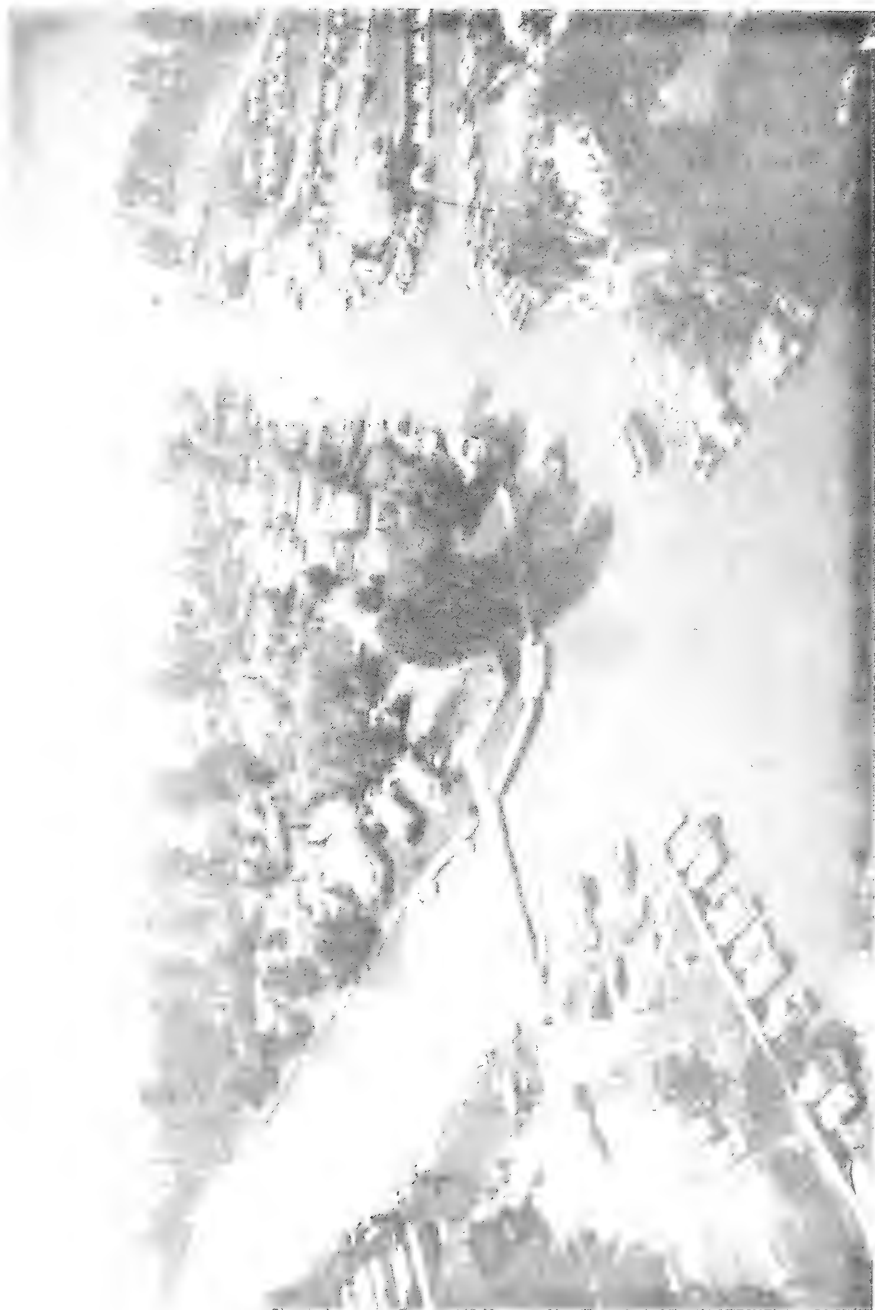
Figure 189. Aerial view of Caseville Harbor, Michigan
