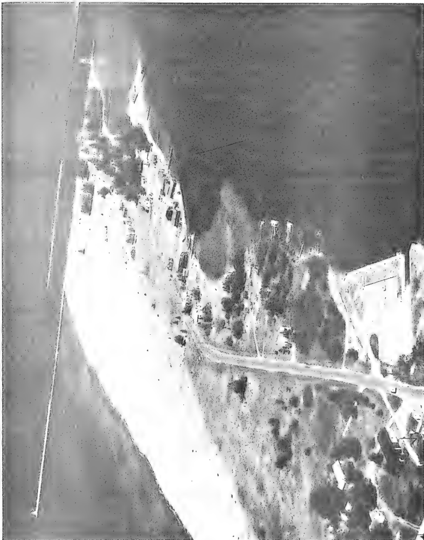
Figure 53. Aerial view of Grand Marais Harbor, Michigan
