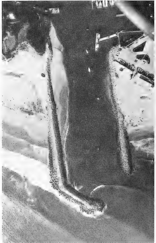
Figure 18. Aerial view of Santa Cruz Harbor jetties
