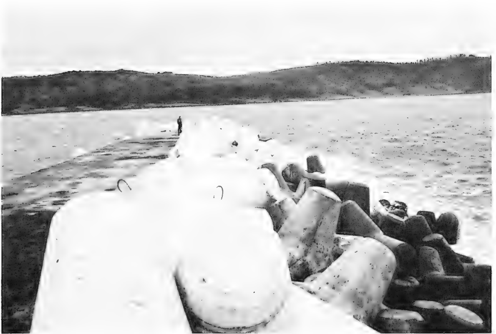
Figure 5. View of tetrapods at head of Crescent City Harbor outer breakwater
