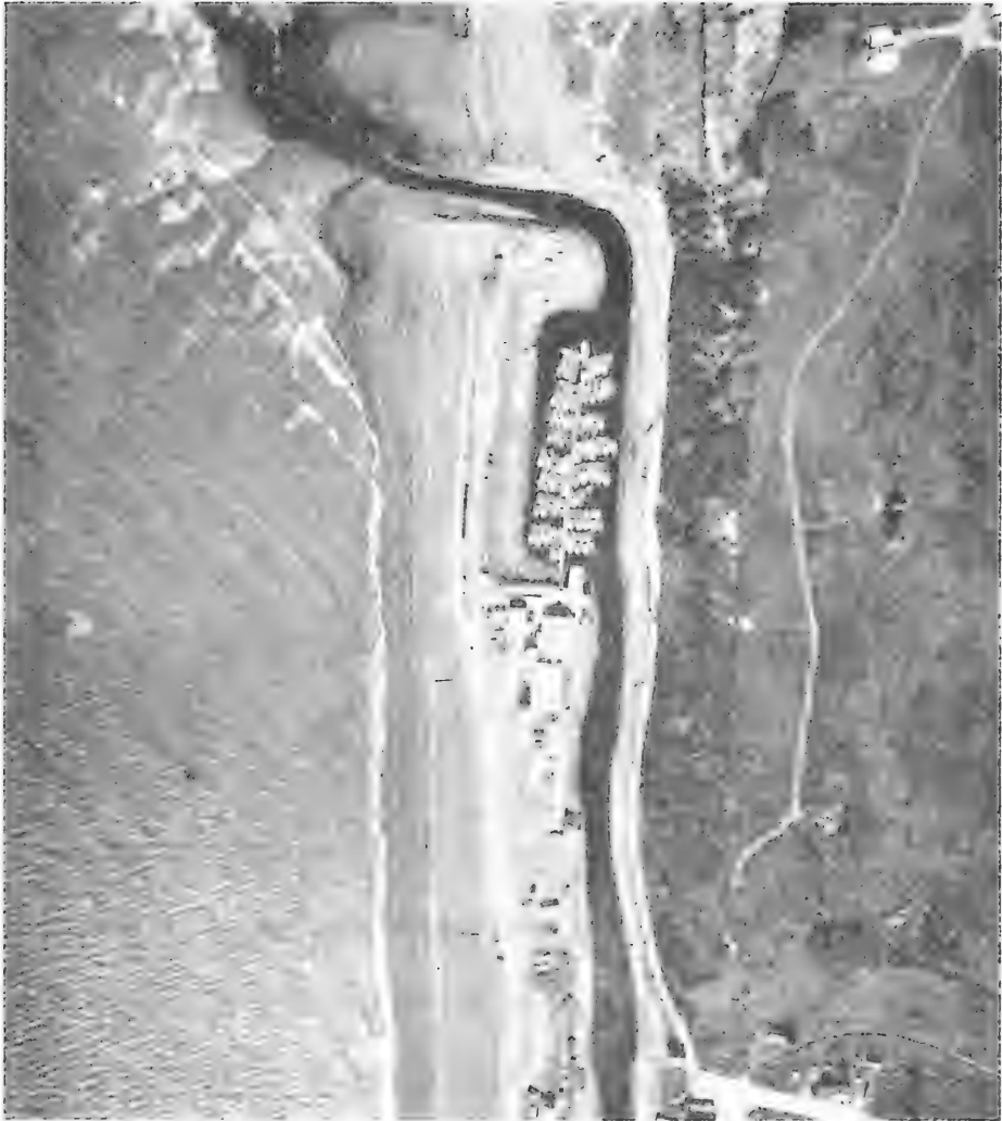
Figure 35. Aerial photograph of Ninilchik Harbor, Alaska, 1980
