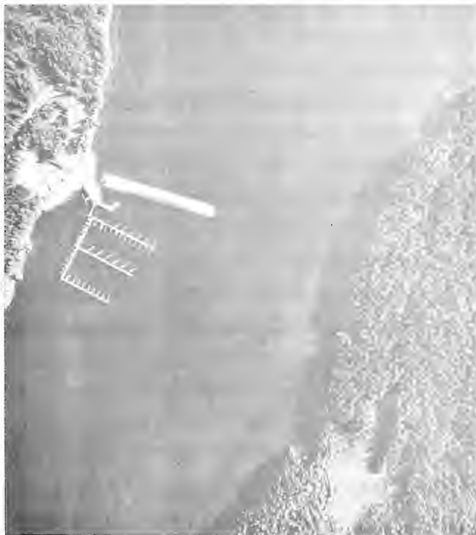
Figure 41. Aerial photograph of Port Lions Harbor, Alaska, 1984
