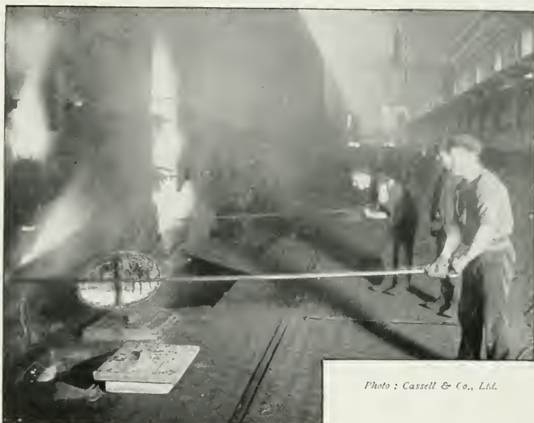
FIG. 4.—A WARM CORNER: DRAWING THE EXHAUSTED CHARGES BY HAND FROM THE RETORT IN THE SOUTH METROPOLITAN GAS COMPANY'S WORKS.
