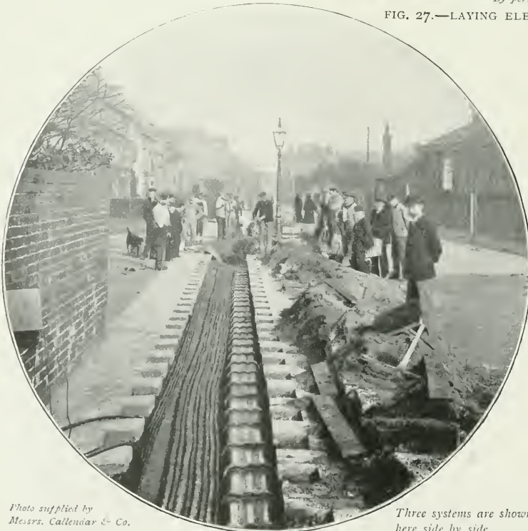
FIG. 28.—LAYING CABLES FOR ELECTRIC LIGHT.
