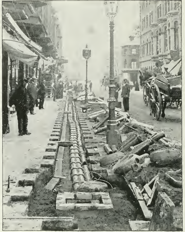
FIG. 27.—LAYING ELECTRIC LIGHT CABLES.
