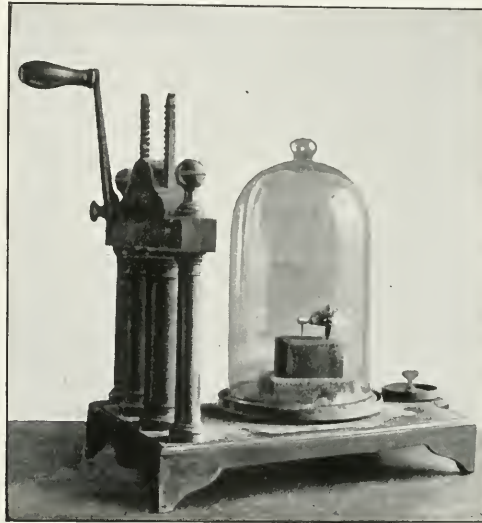
FIG. 1.—BELL UNDER AIR PUMP.
