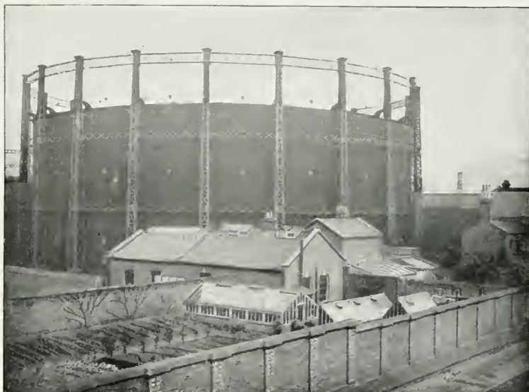
FIG. I.—GASOMETER AT BATTERSEA PARK.
