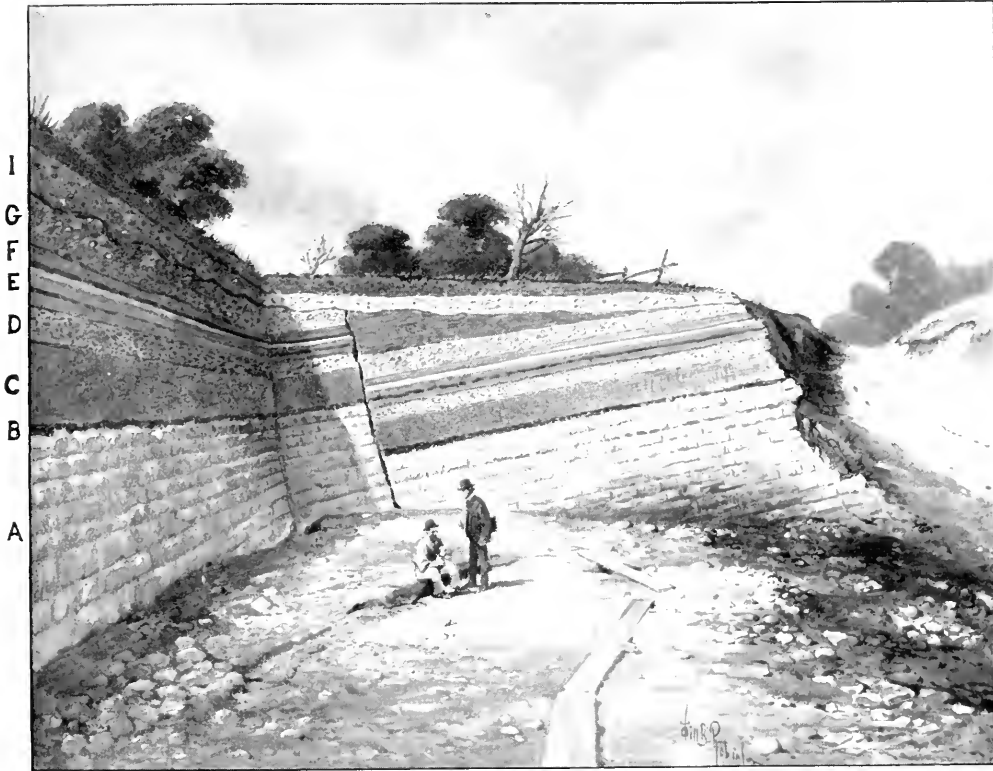
FIG. 2.—SHOWING THE STRATA MET WITH IN A QUARRY.
