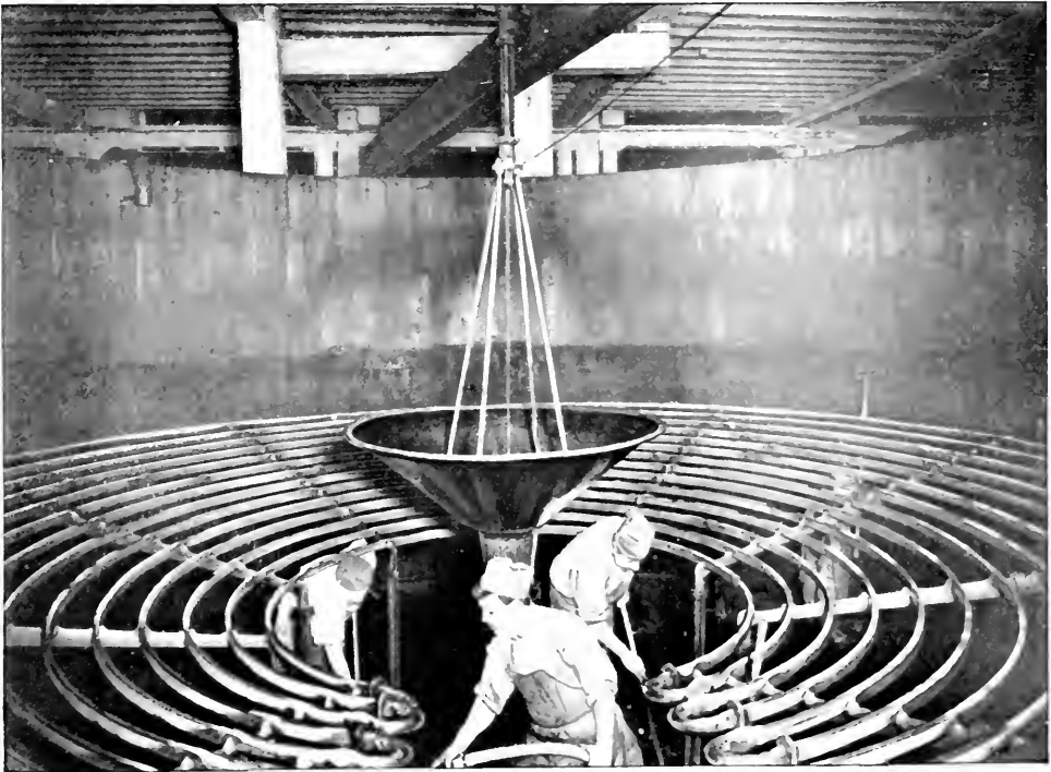
FIG. 6.—CLEANING OUT THE FERMENTING VAT. From a photograph taken in Messrs. Meux & Co's Brewery.
