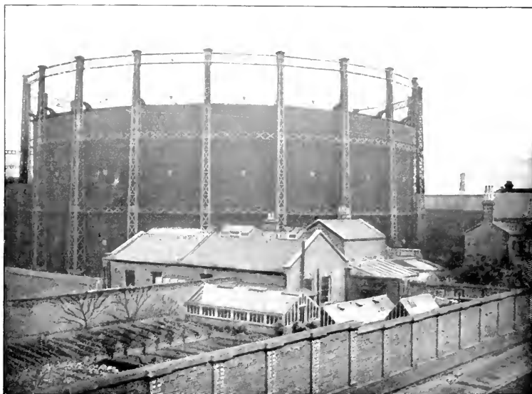
FIG. I.—GASOMETER AT BATTERSEA PARK.
