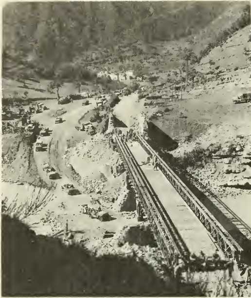
TRUCK CROSSING TREADWAY BRIDGE HASTILY CONSTRUCTED BY ENGINEERS IN APENNINES
