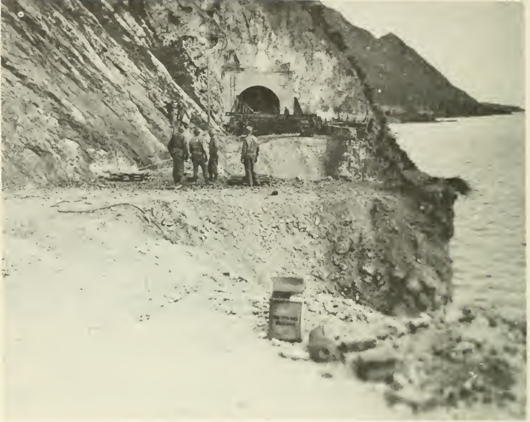
ENGINEERS REPAIRING APPROACH TO TUNNEL, LAKE GARDA
