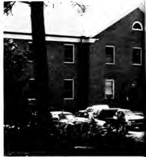
Queen Anne Hall, the first in the new wave of construction, currently houses all women boarding students.
