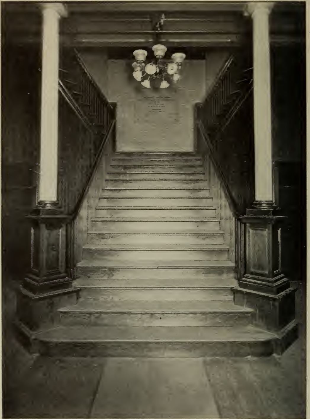
MAIN STAIRWAY, MACHINERY BUILDING.
