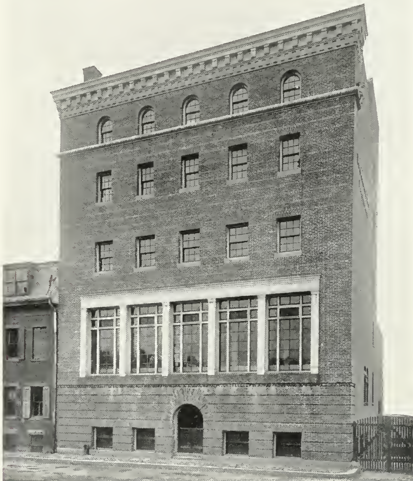
NEWCOMB STREET BUILDING Connected with Building on previous page
