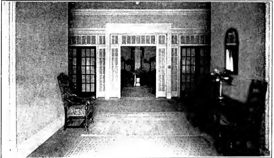
HALLWAY IN ADMINISTRATION BUILDING
