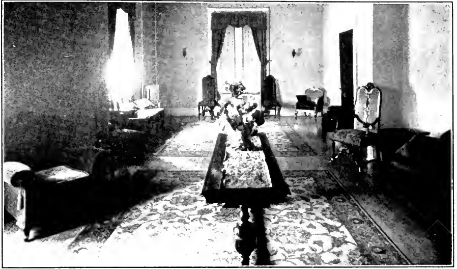
DRAWING ROOM, ADMINISTRATION BUILDING
