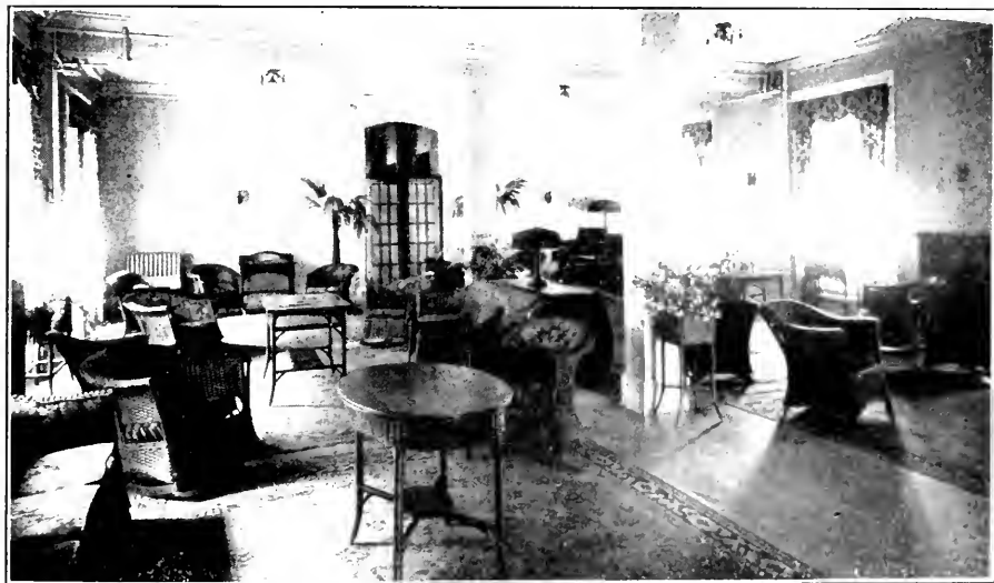
SOCIAL HALL, ADMINISTRATION BUILDING
