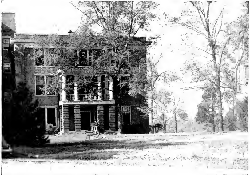
MATTHEW S. DAVIS MEMORIAL BUILDING
