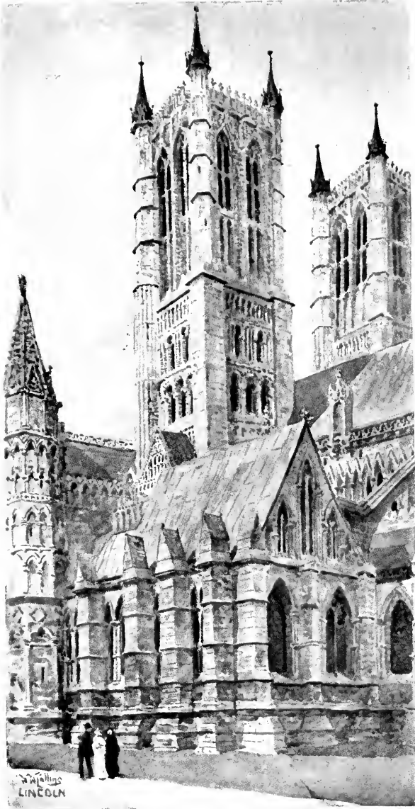
LINCOLN THE WEST TOWERS
